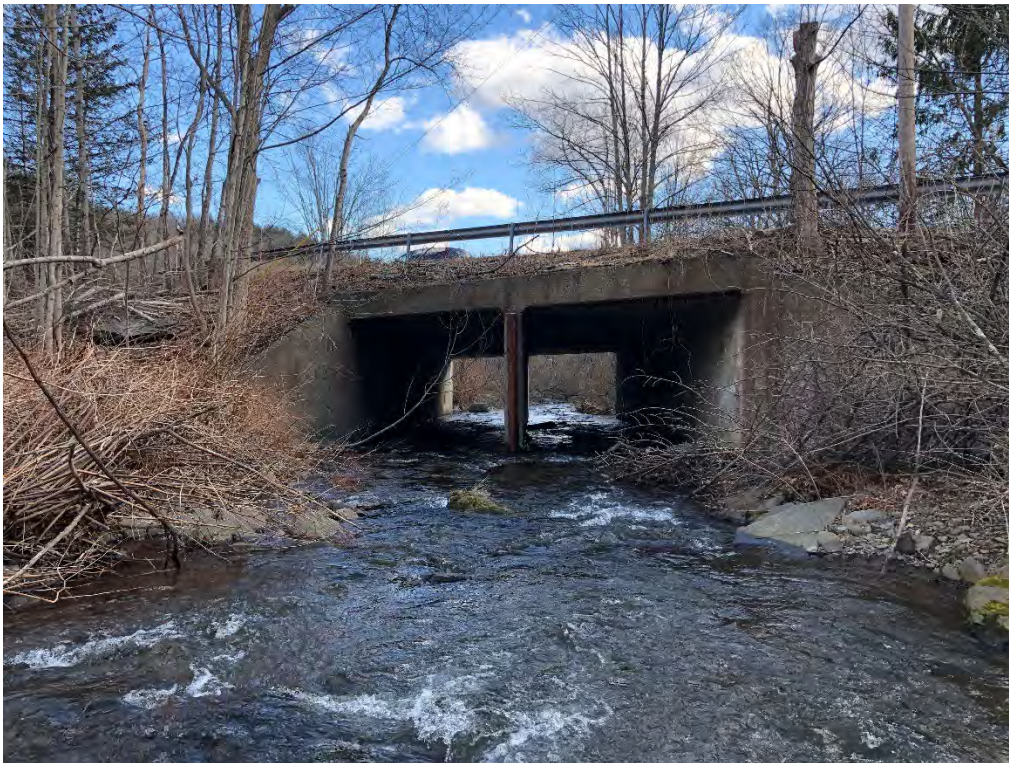
Figure 4-41: Looking downstream at the Elm Street culvert over Birch Creek
