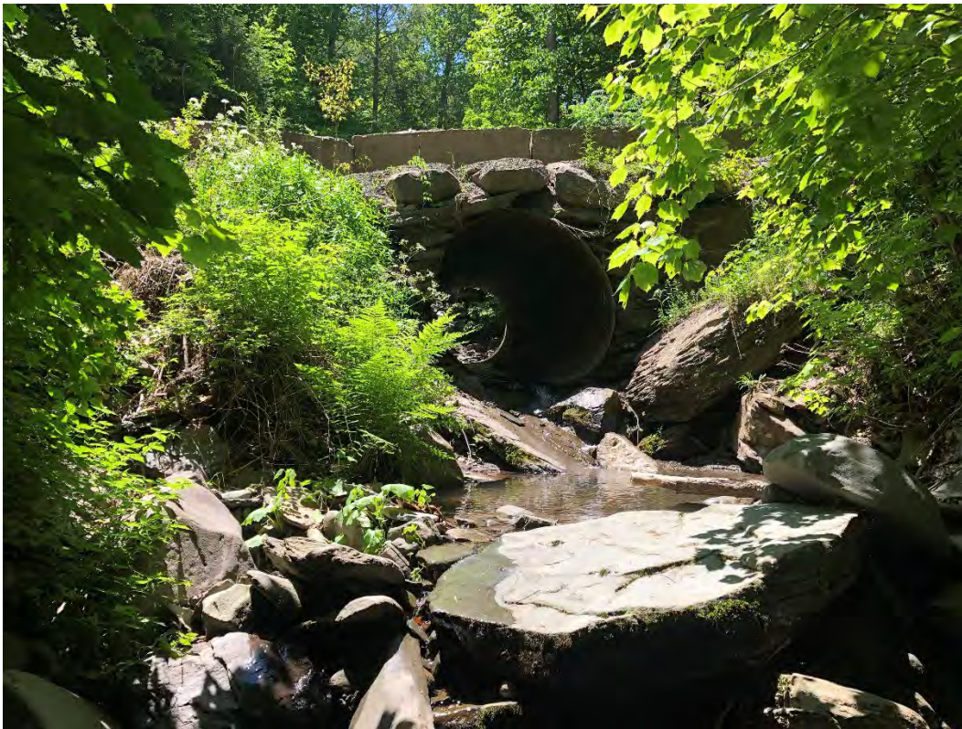
Figure 4-44: Outlet and tailwater of Station Road culvert at Woodchuck Hollow
