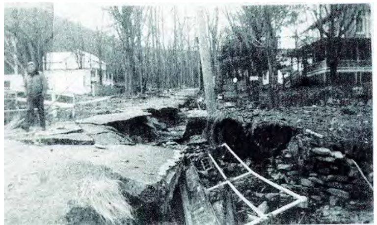
Figure 3-1: Photos depicting flooding damage in Pine Hill due to the Rainmaker flood event in November 1950. Photo Sources: Catskill Mountain News
