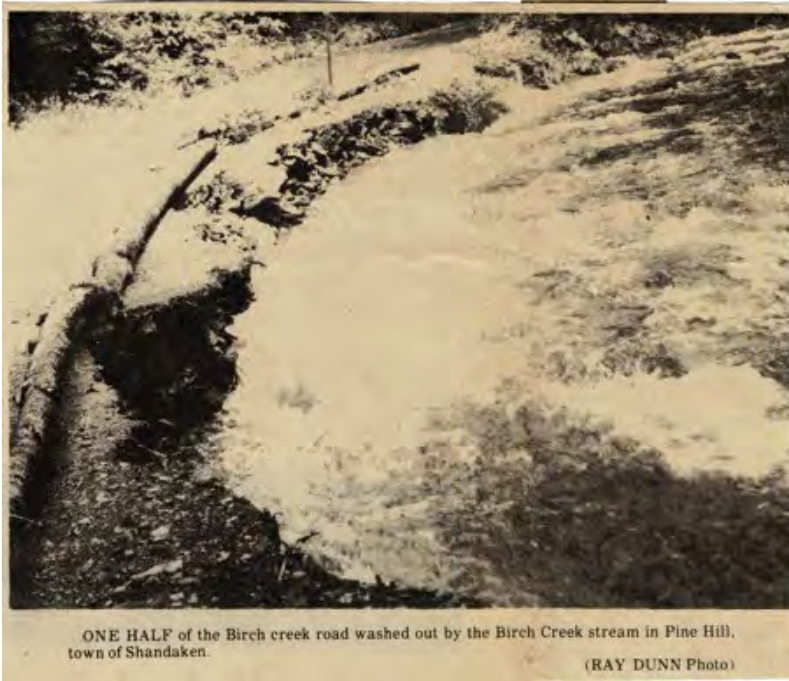
Figure 3-2: A photo depicting flood damage within the hamlet of Pine Hill on Birch Creek Road during the July 1973 event. Photo Source: Catskill Mountain News
