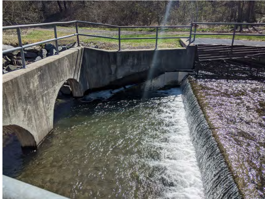
Figure 4-42: Dam, old road crossing, and intake for Belleayre Day Use Area
