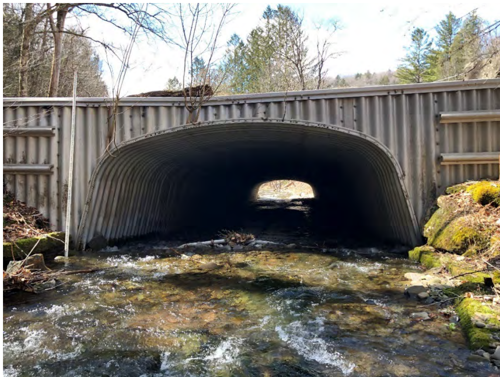
Figure 4-40: Looking downstream at Birch Creek Road culvert over Birch Creek
