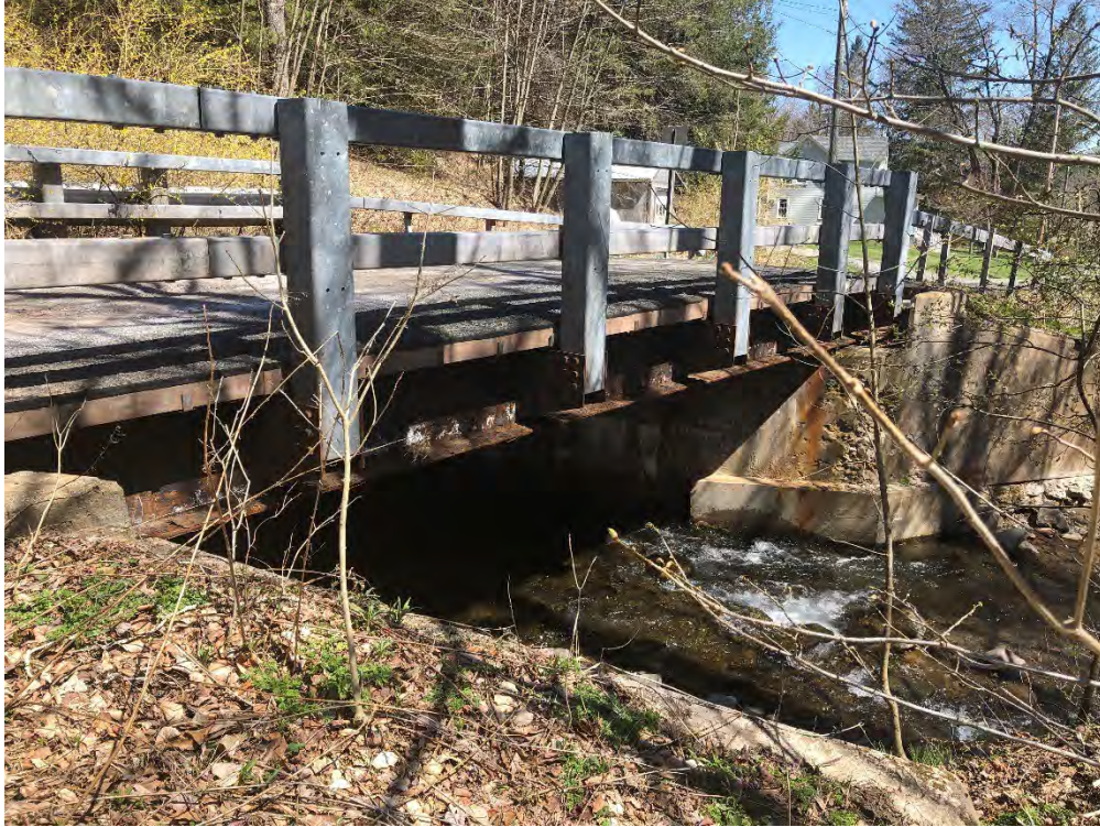
Figure 4-3: Outlet of county bridge over Alton Creek
