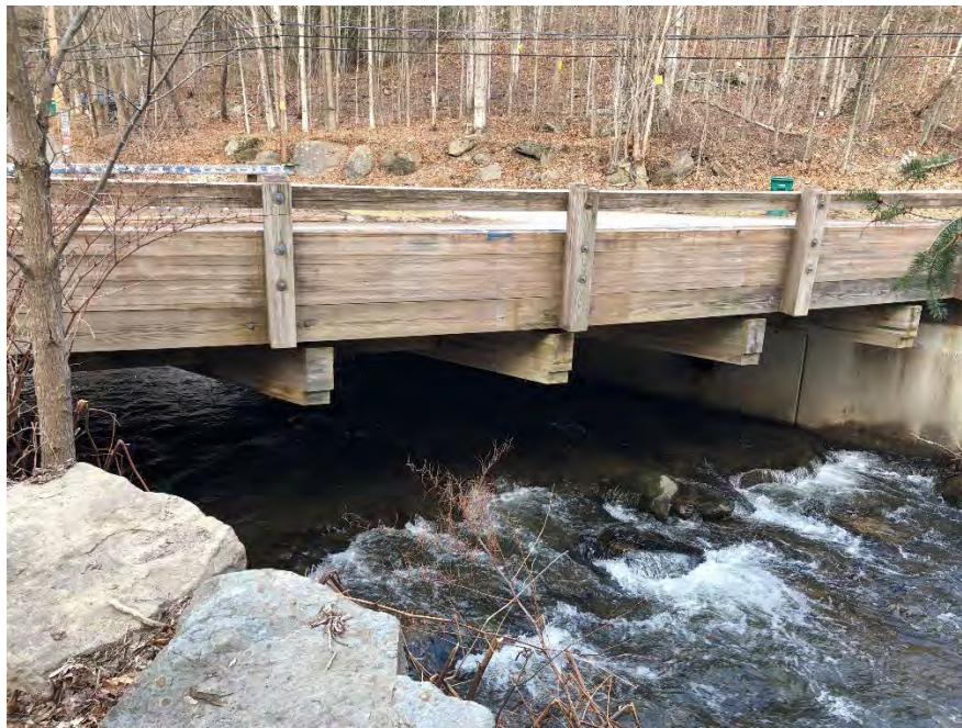
Figure 4-34: Looking downstream at the lower Main Street crossing over Birch Creek
