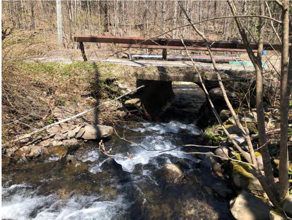
Figure 4-20: Inlet of culvert crossing Alton Creek
