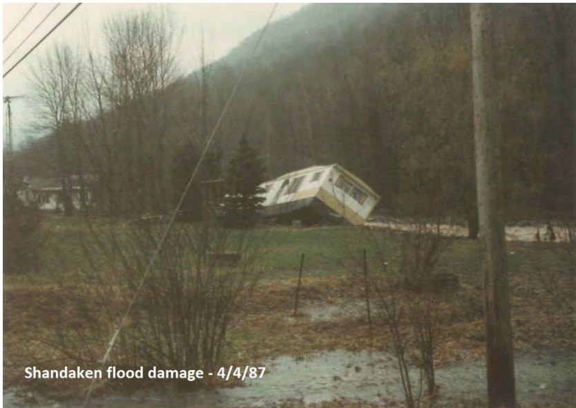
Figure 3-4: A photo depicting flood damage within the hamlet of Pine Hill during the April 1987 event. Photo Source: Aaron Bennett, NYCDEP
