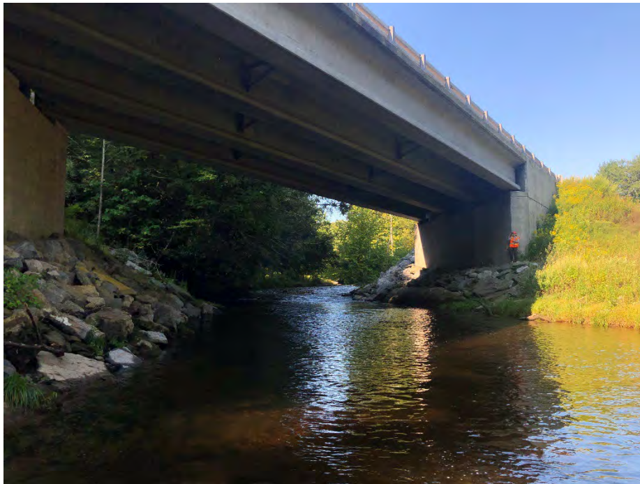
Figure 4-2: Downstream outlet opening of the State Route 55 bridge
