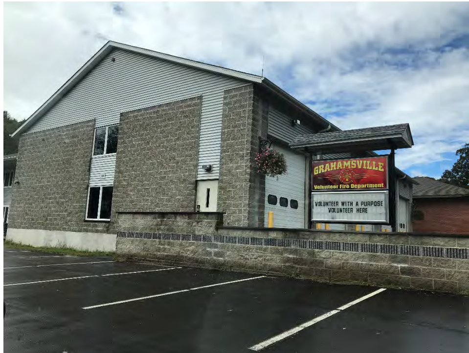
Figure 2-8: Grahamsville Volunteer Fire Department, a critical facility
