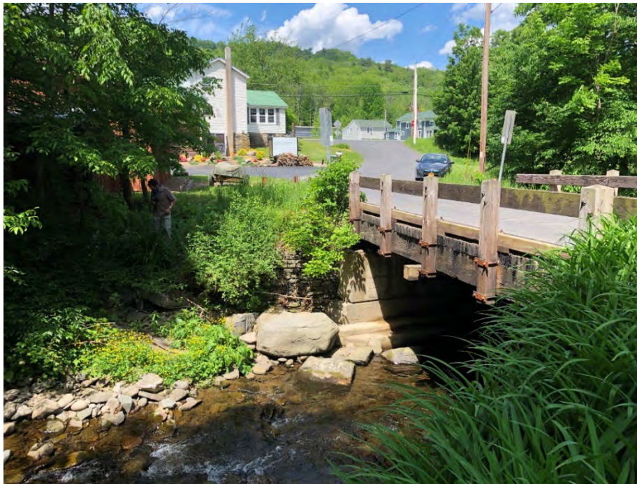
Figure 4-15: Looking downstream at the Hilltop Road bridge inlet over Chestnut Creek
