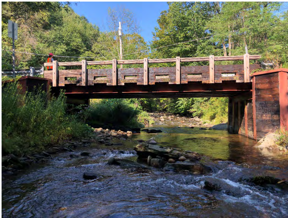
Figure 4-16: Looking upstream at the Clark Road bridge
