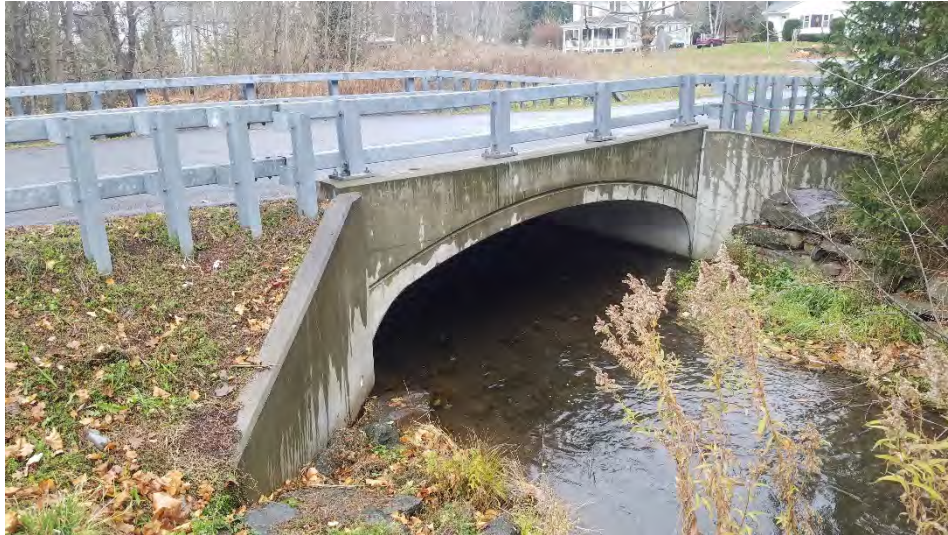
Figure 4-1: Roosevelt Avenue over WBDR (looking downstream at culvert inlet)
