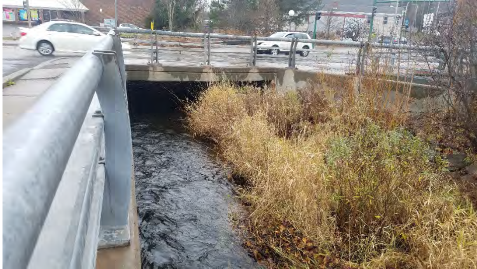
Figure 4-3: Main Street culvert over WBDR (looking downstream at culvert inlet)
