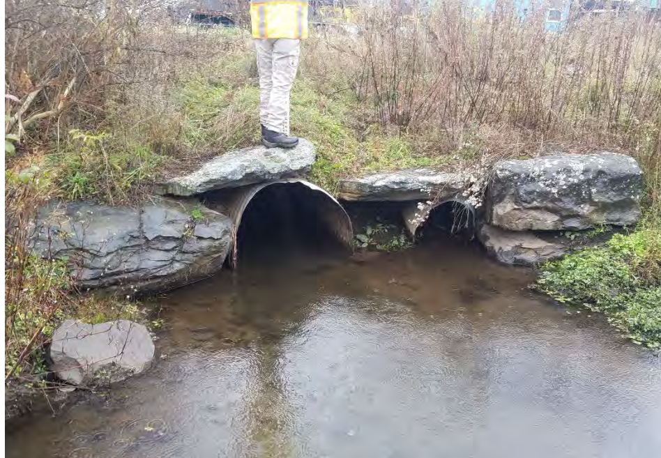
Figure 4-16: Graham Drive culvert outlets (looking upstream)
