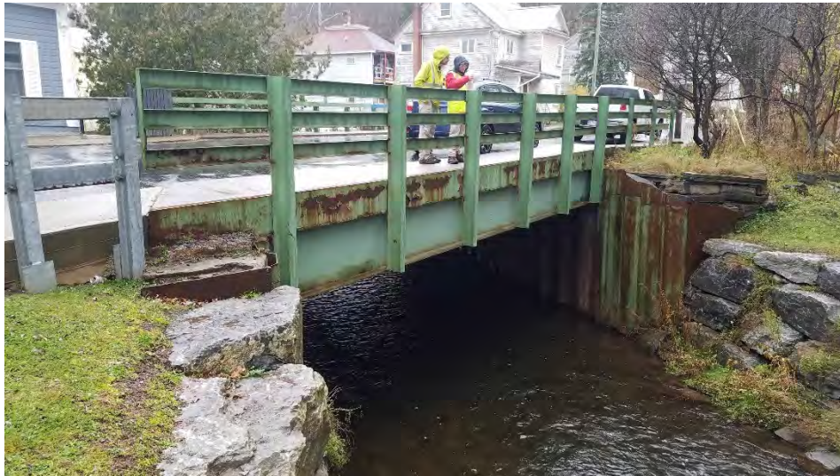
Figure 4-19: Cornell Avenue bridge upstream opening (looking downstream)
