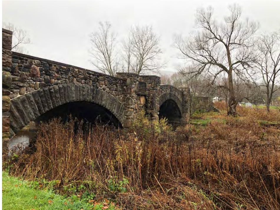
Figure 4-27: County Route 18 downstream bridge face
