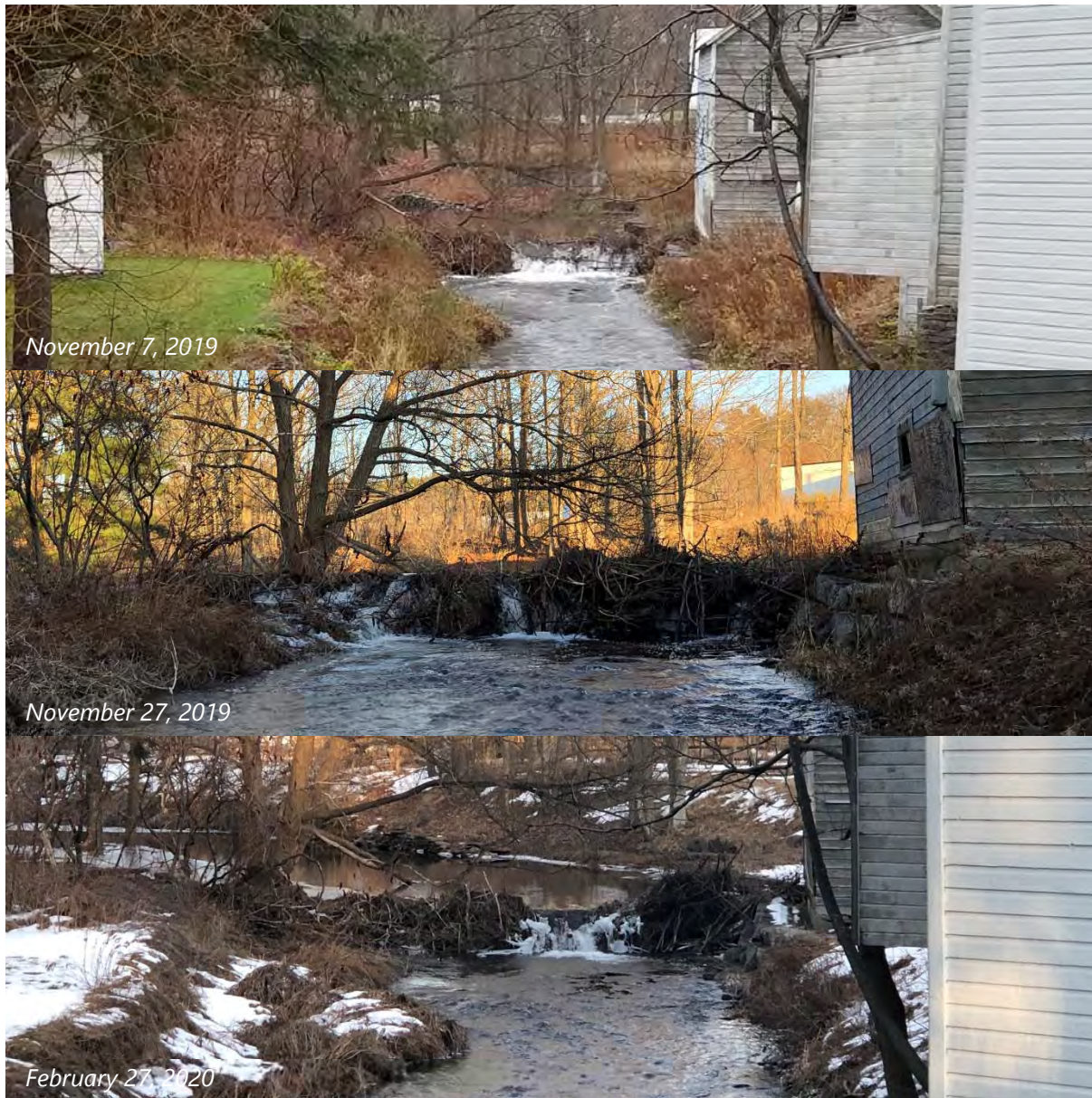
Figure 4-42: Photos of dam remnants taken at three separate occasions. Middle image shows beaver dam built across the top of the dam.
