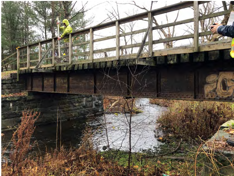
Figure 4-13: Upstream rail trail bridge face (looking downstream)
