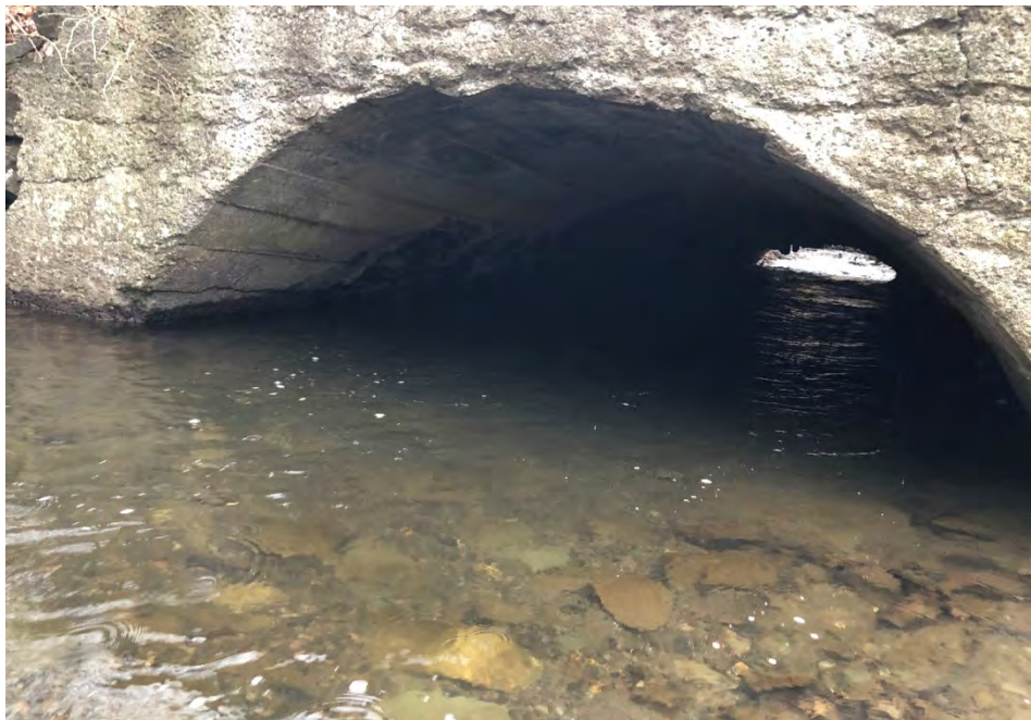
Figure 4-6: South Street culvert outlet (looking upstream through culvert)
