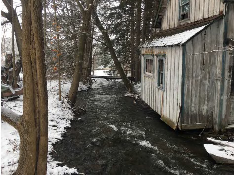
Figure 4-36: Structures potentially obstructing flows on the WBDR and lack of well-established riparian buffer zone
