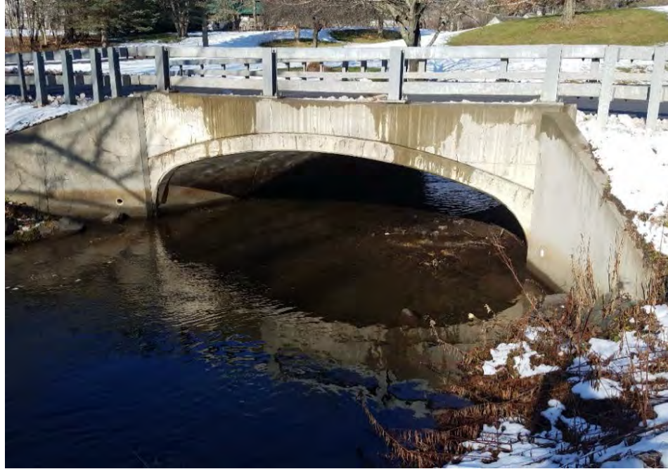
Figure 4-14: Railroad Avenue outlet (looking downstream)
