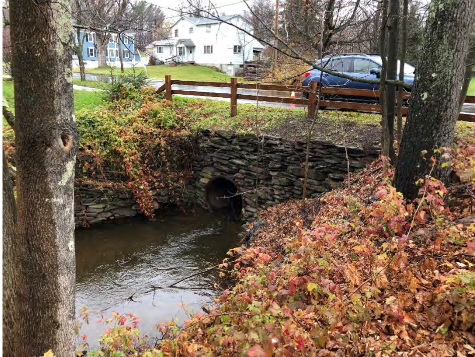
Figure 4-21: Maple Avenue culvert outlet (looking upstream at downstream headwall)
