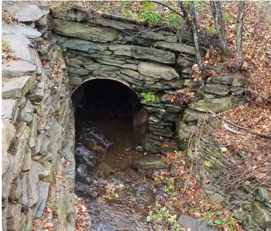
Figure 4-20: Maple Avenue culvert inlet (looking downstream at upstream headwall)
