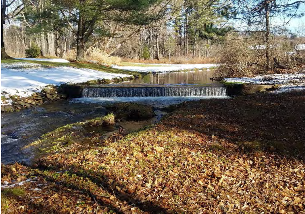
Figure 4-43: Low-head dam on the WBDR (looking upstream)
