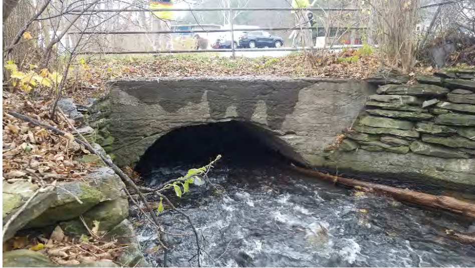
Figure 4-5: South Street culvert inlet (looking downstream at upstream headwall)
