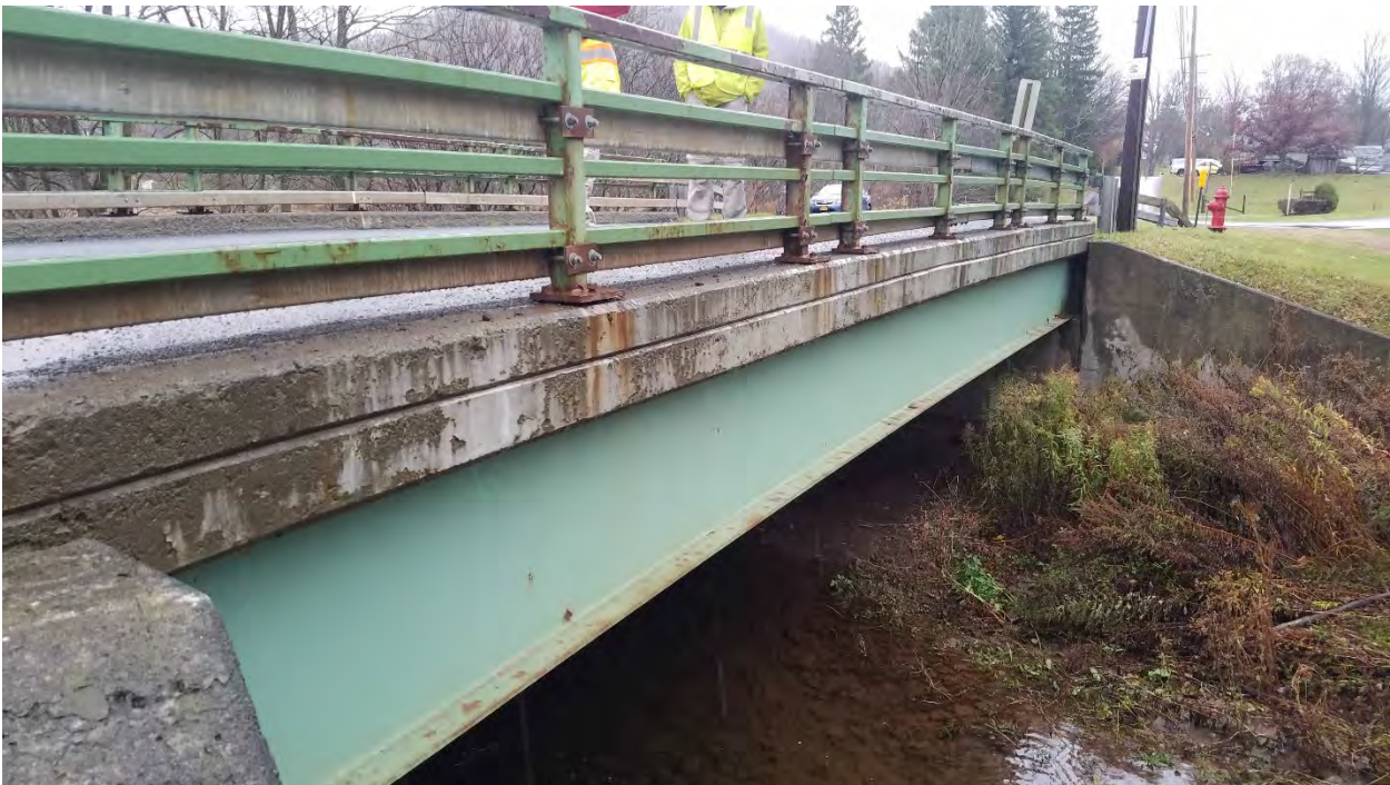
Figure 4-25: Downstream bridge face
