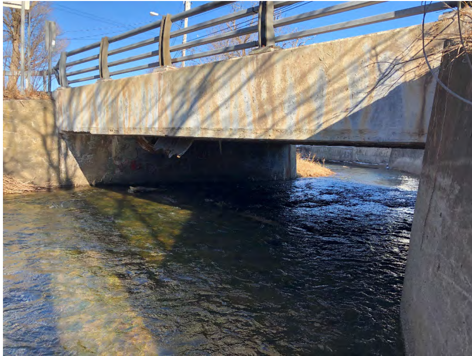
Figure 4-10 NYS Route 30 Bridge over the Bear Kill in Grand Gorge
