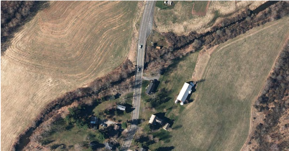
Figure 4-4 NYS Route 30 Bridge in Roxbury, New York, over EBDR
