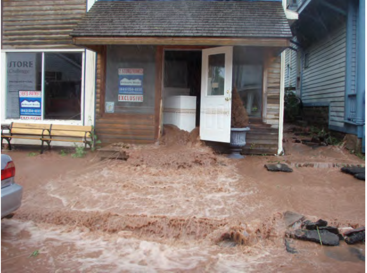
Figure 4-36 Floodwaters from Vega Mountain Stream Flowing Through a Building that is Located on the Northern Corner of the Vega Mountain Road /NYS Route 30 Intersection
