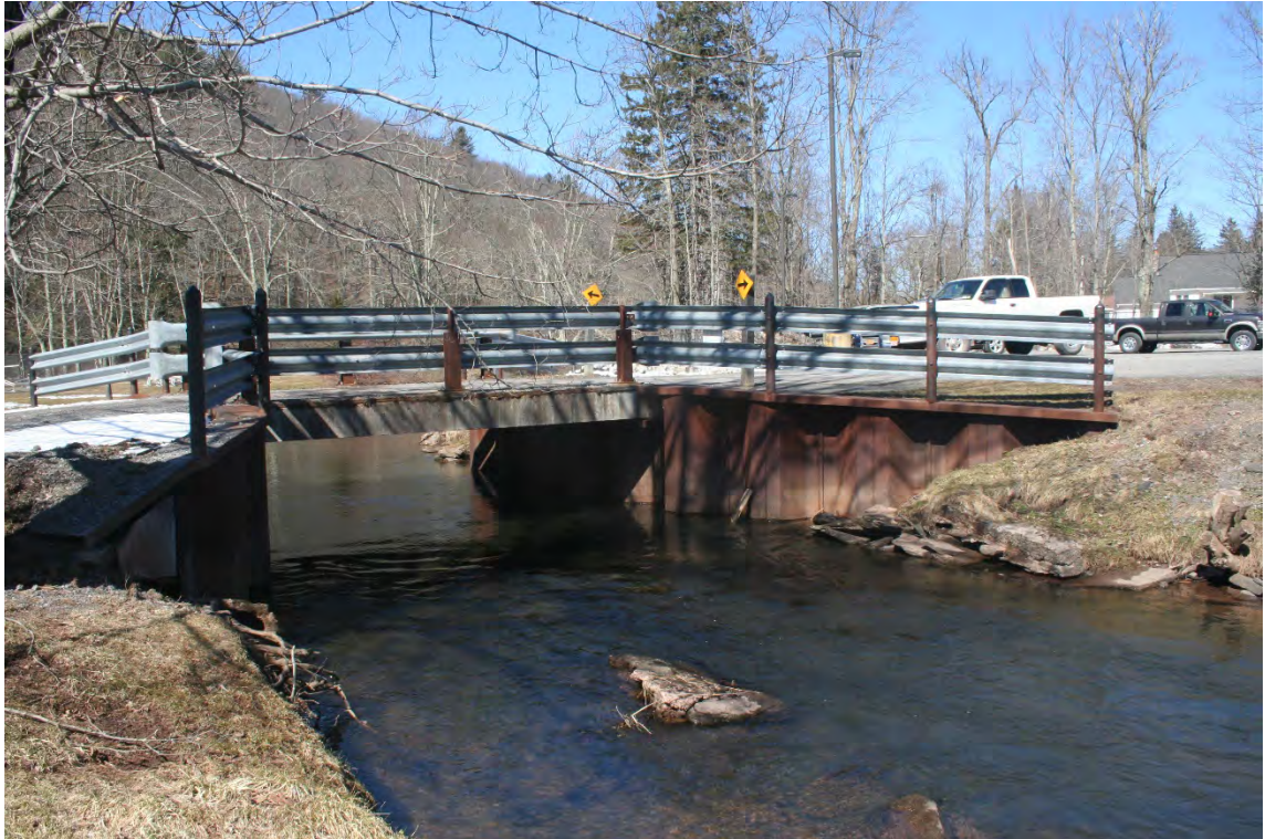
Figure 4-5 Bridge Behind Roxbury School over EBDR
