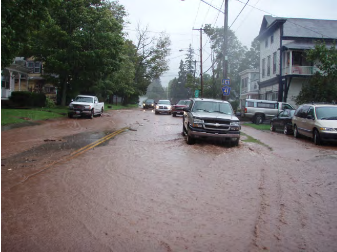
Figure 3-5 (Facing South on NYS Route 30 near Roxbury Fire Department Building) Vega Mountain Stream Floodwaters Traveling across the Backyards of Homes North of Route 30 and Flooding Main Street
