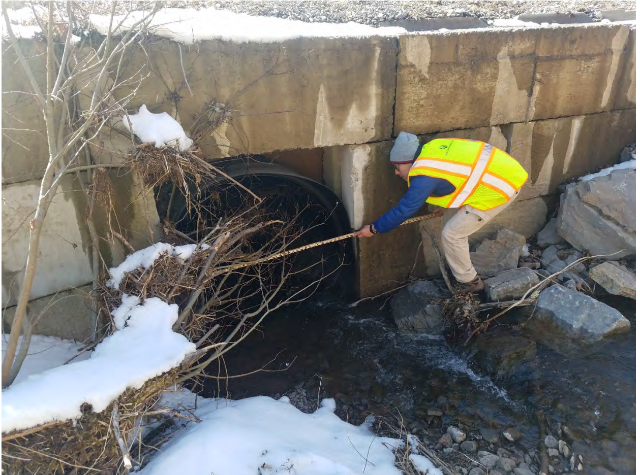
Figure 4-38 Inlet of the Johnson Road Culvert carrying Vega Mountain Stream
