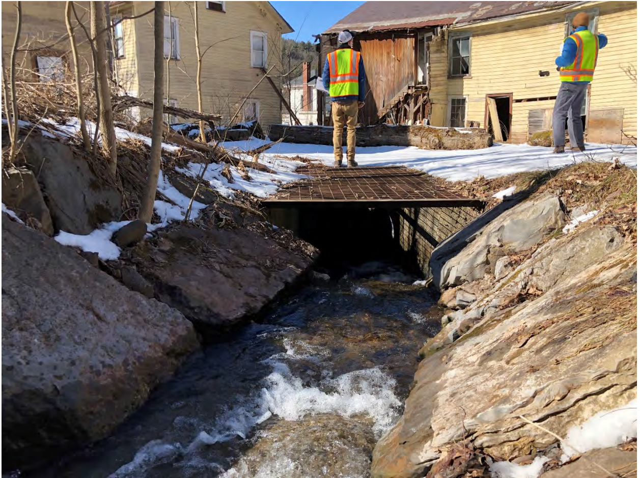
Figure 4-33 Inlet Structure to Pipe Flowing under NYS Route 30, Vega Mountain Stream
