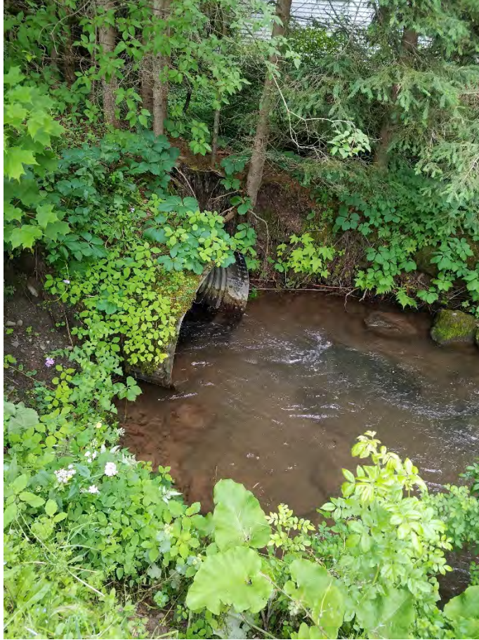
Figure 4-34 Outlet Culvert of Pipe System under NYS Route 30
