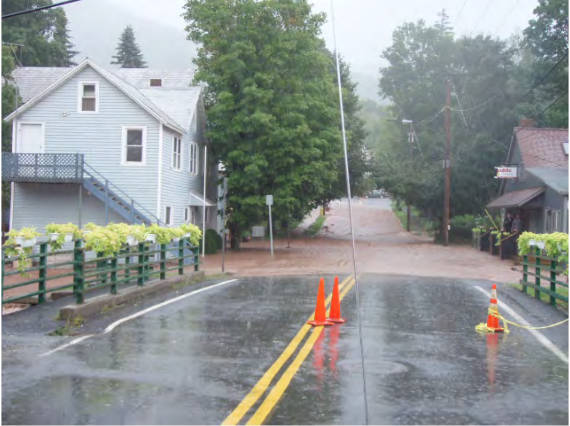
Figure 4-6 Bridge Street Bridge over EBDR during Tropical Storm Irene
