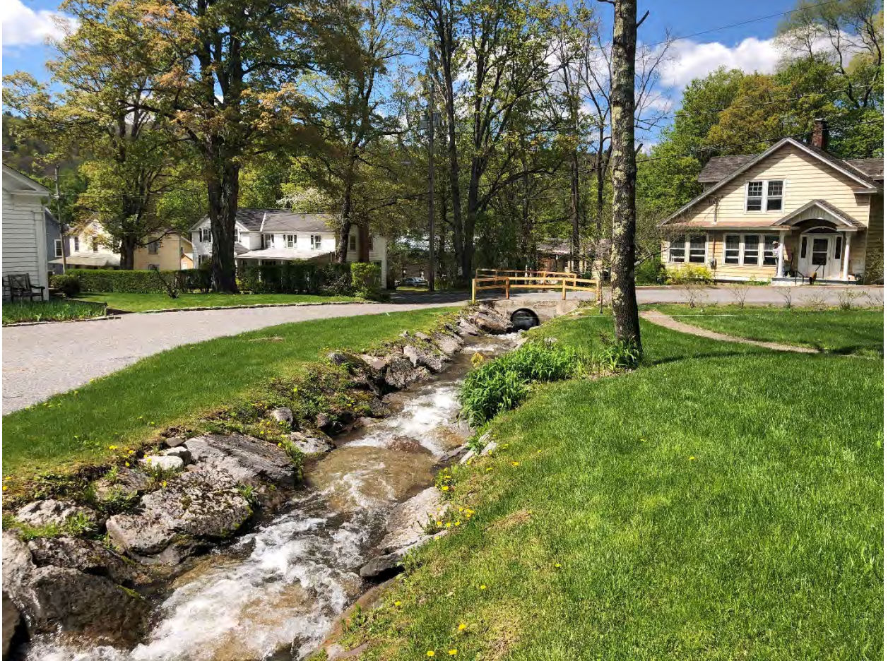
Figure 4-35 Culvert Carrying Vega Mountain Road (Looking Downstream)
