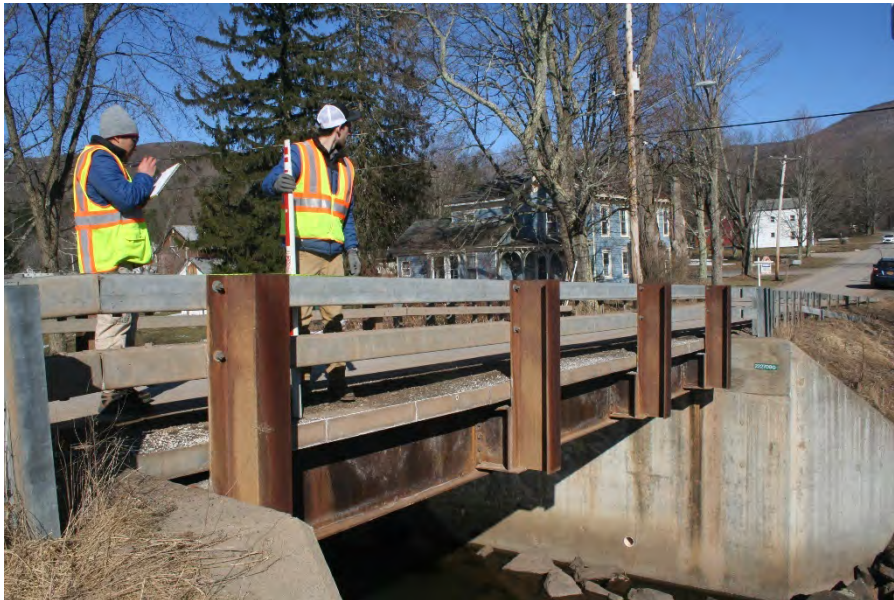
Figure 4-3 North Montgomery Road Bridge over EBDR
