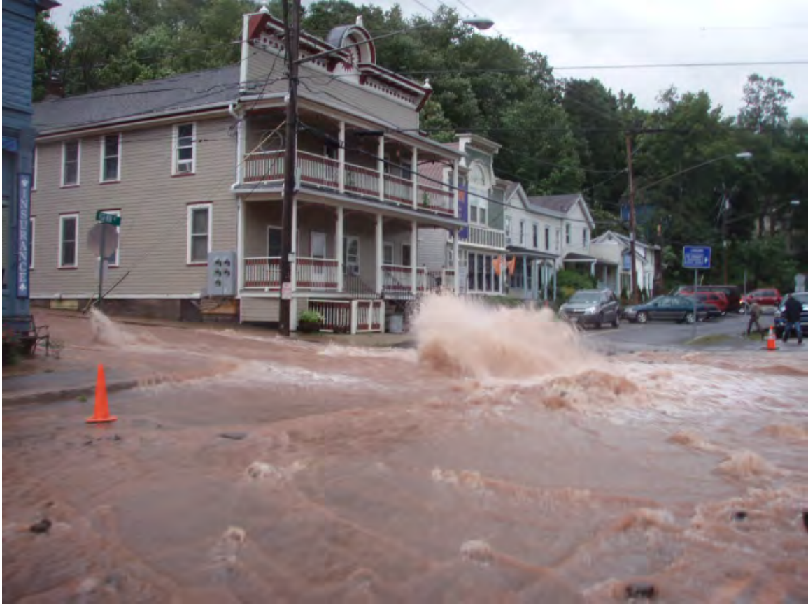
Figure 3-4 High-Velocity Floodwaters Traveling Down Vega Mountain Road toward NYS Route 30; Energy Dissipation Causes a Hydraulic Jump at Intersection
