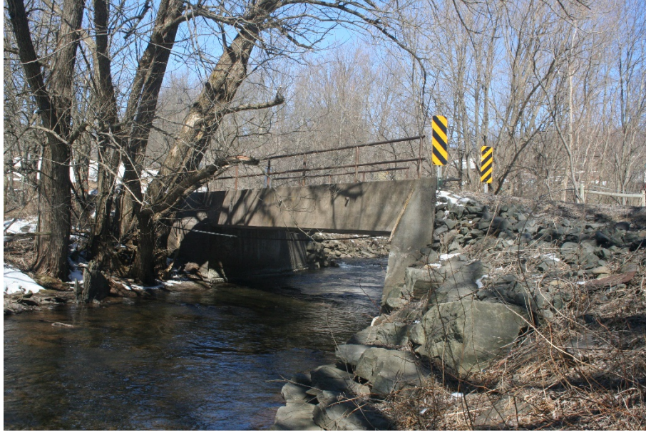
Figure 5-15: Ursum Way bridge over Vly Creek. Looking upstream from left bank.
