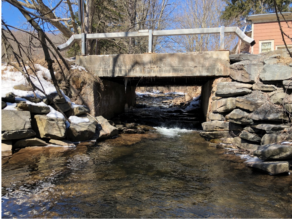
Figure 5-9: County Route 3 crossing of Brownell Creek. View looking upstream.
