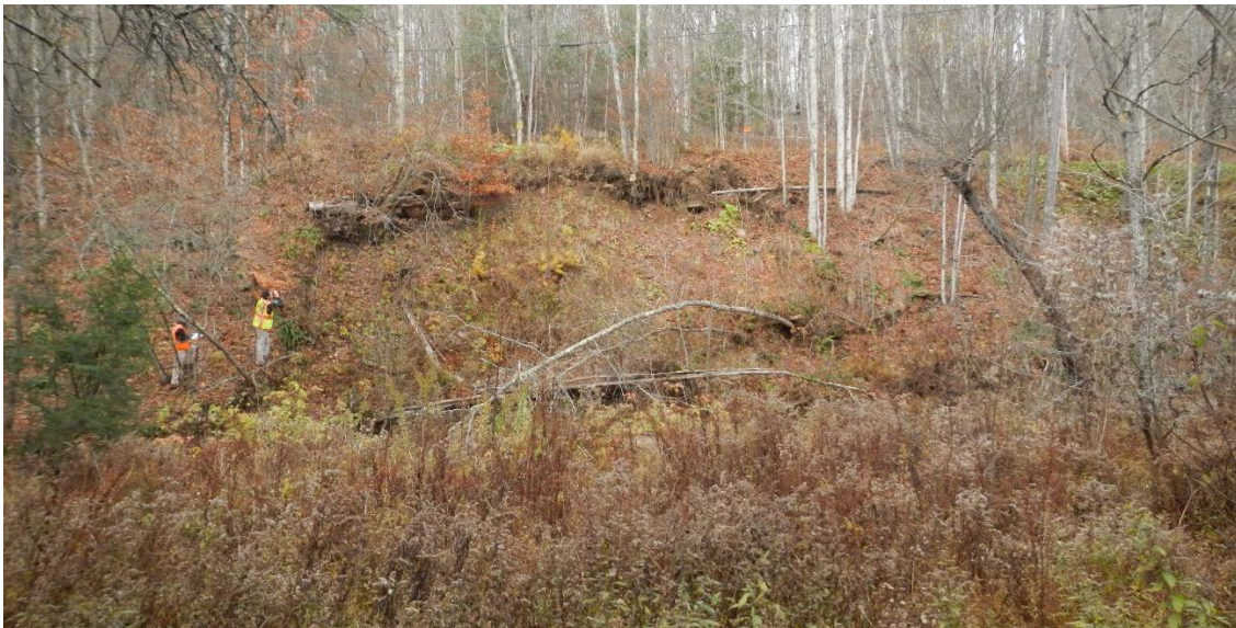
Figure 5-20: Bank failure along Elk Creek Road. Photo taken from opposite bank of Elk Creek.
