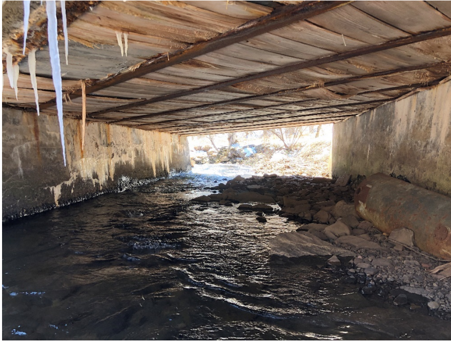
Figure 5-7: County Route 1 culvert over Brownell Creek. View inside culvert, looking downstream.
