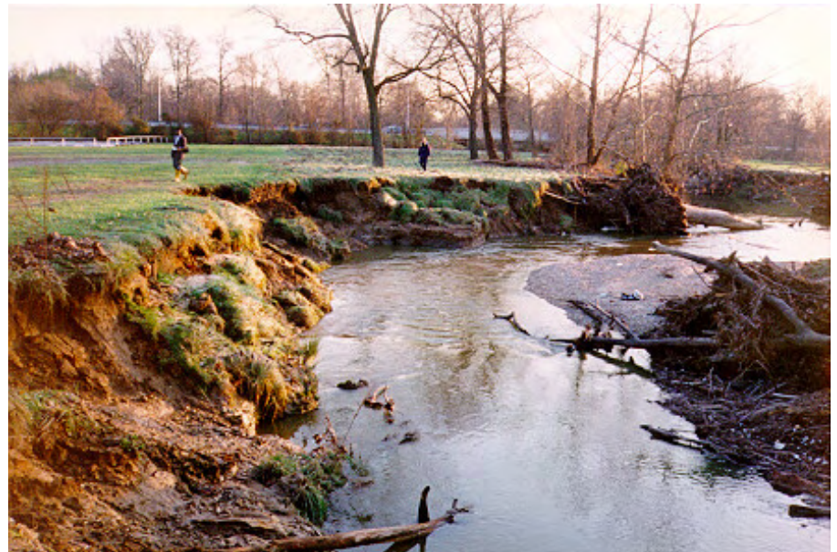
Figure 8. Example of eroded stream banks. There is no vegetation and few roots along the stream to provide structural stabilization. The erosive force of the water cuts the banks and carries sediment downstream, thereby degrading water quality.
