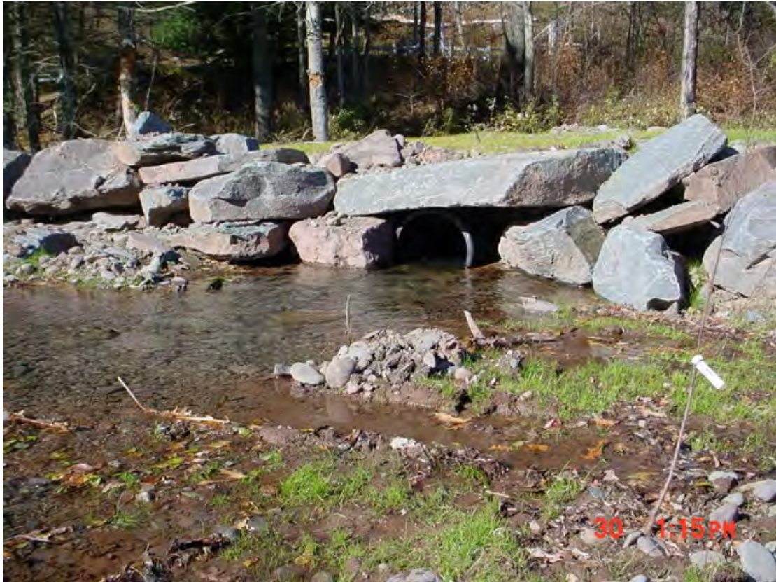
Figure E1 Small tributary confluence through culvert
