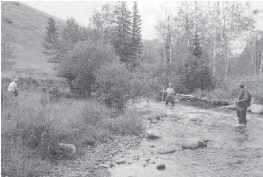
Figure 50. Measuring along the channel centerline and staking.
