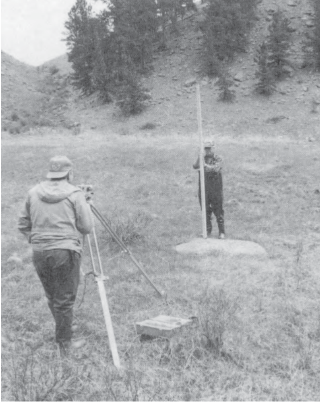
Figure 34. Shooting the elevation of the benchmark.
