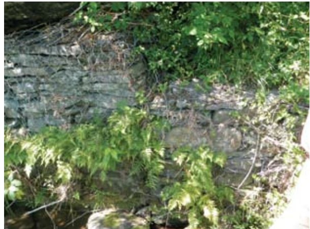
Stone gabion revetment on right bank (P7190130)
