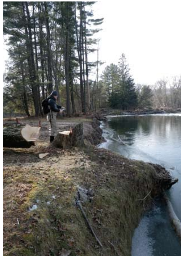
Erosion on the left bank near Station 28080. (IMGP2304)
