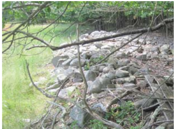
Berm along left bank (B304)
