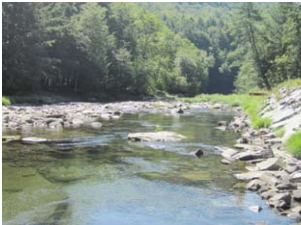
Exposed bedrock providing grade control (A260)
