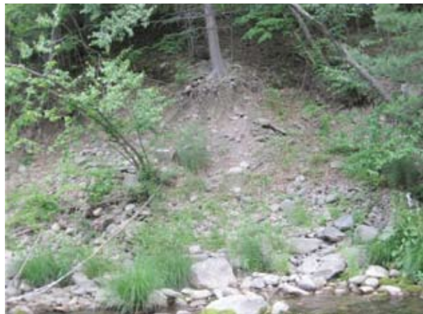
Stabilizing slope failure on right bank (A334)
