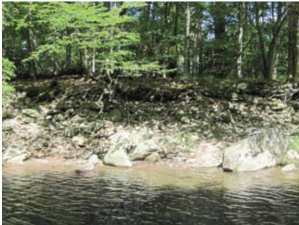
Erosion on left bank (B319)
