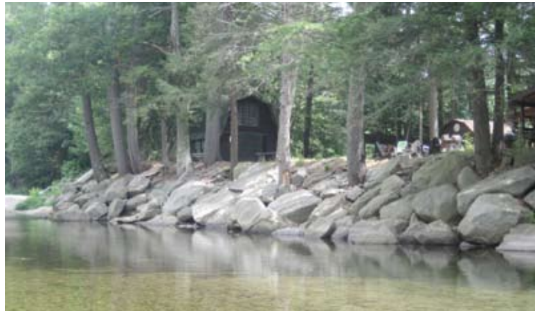
Looking upstream, large stacked revetment on left bank (B394)
