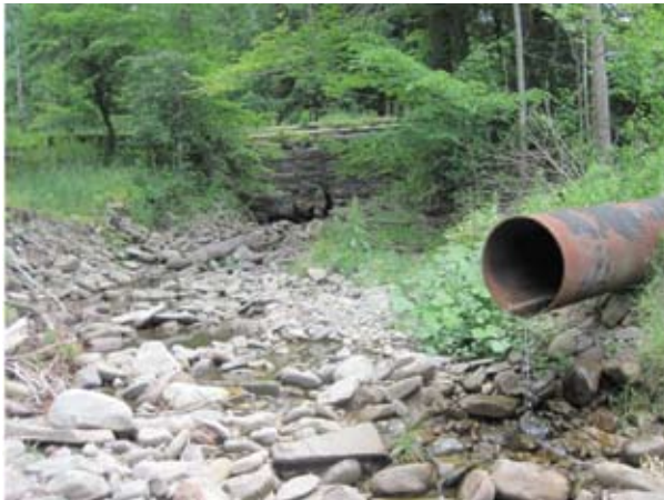
Drainage pipe from Wildcat Road (A313)
