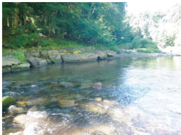
Placed quarry rock forming grade control (P7290125)
