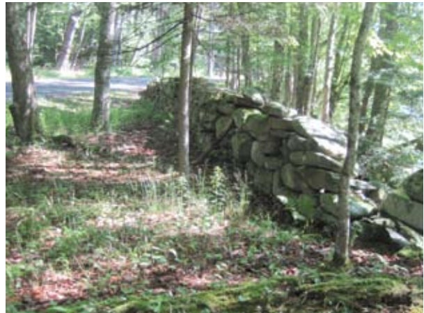
Actively maintained berm on right floodplain (A237)
