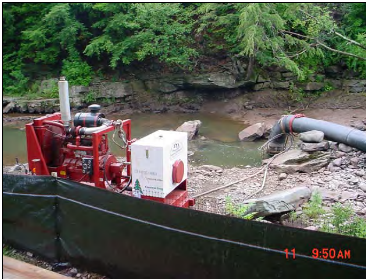
Figure 7 - Dewatering equipment Installed on Site
