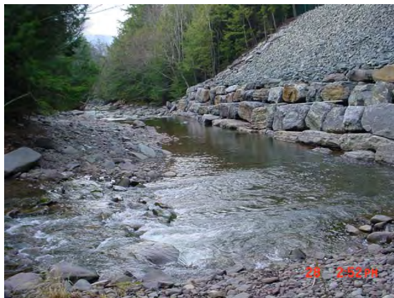
Rockery Wall on Gooseberry Creek.
