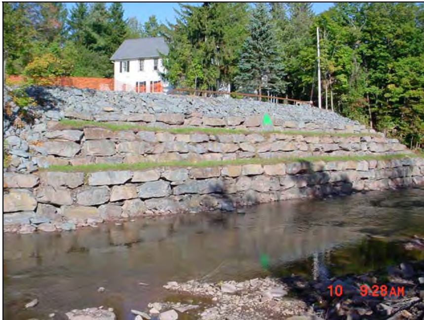
Figure 6 - Completed Embankment Repair
