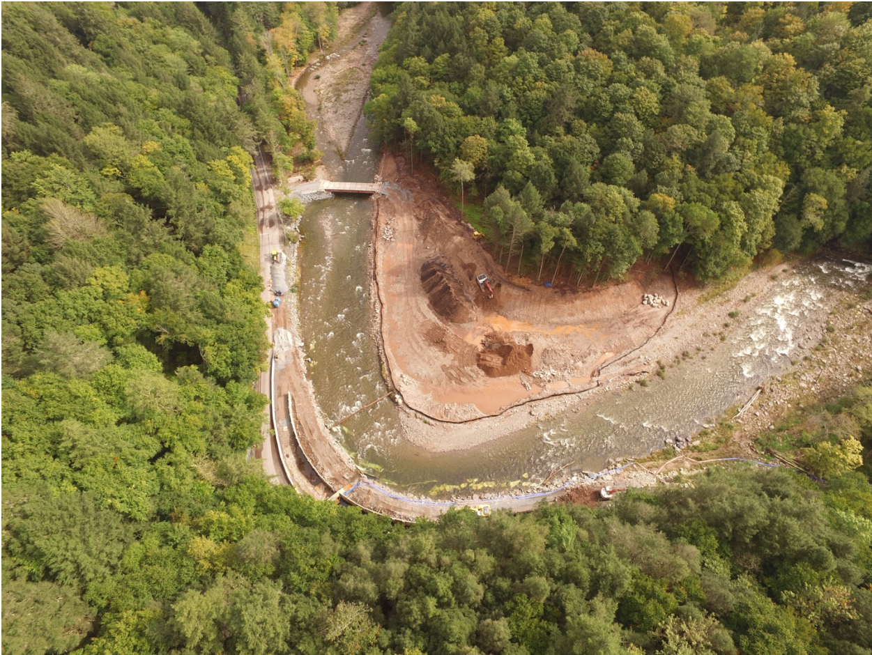
FLOOD HAZARD MITIGATION IMPLEMENTATION PROJECT AT COUNTY ROAD 47 ULSTER COUNTY 2018
