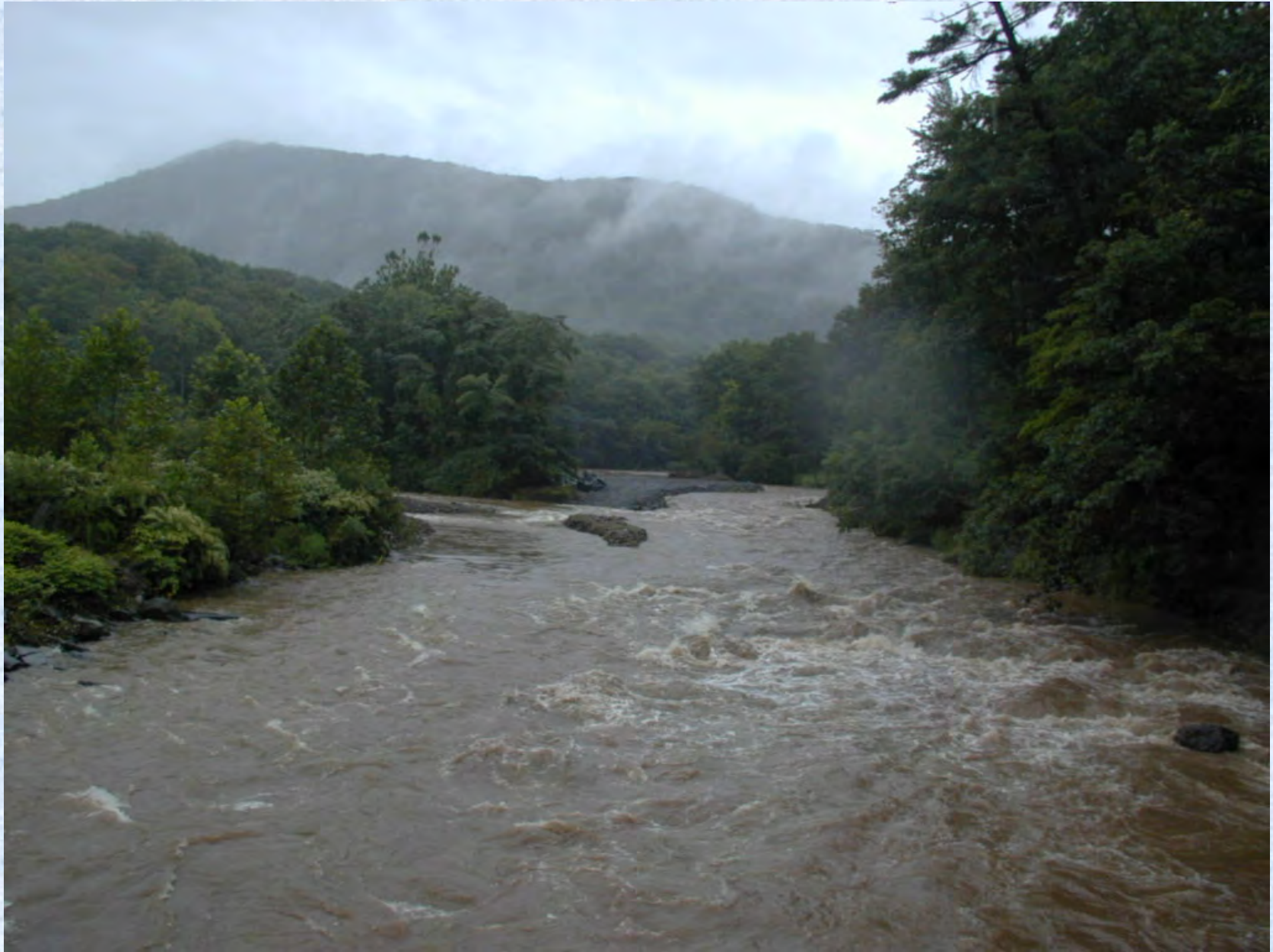
View from Woodland Valley Bridge
