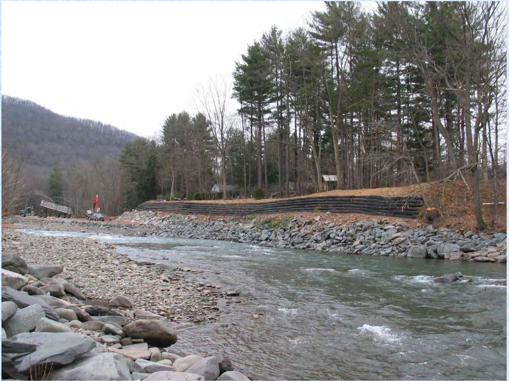
Vegetated Reinforced Soil Slope
