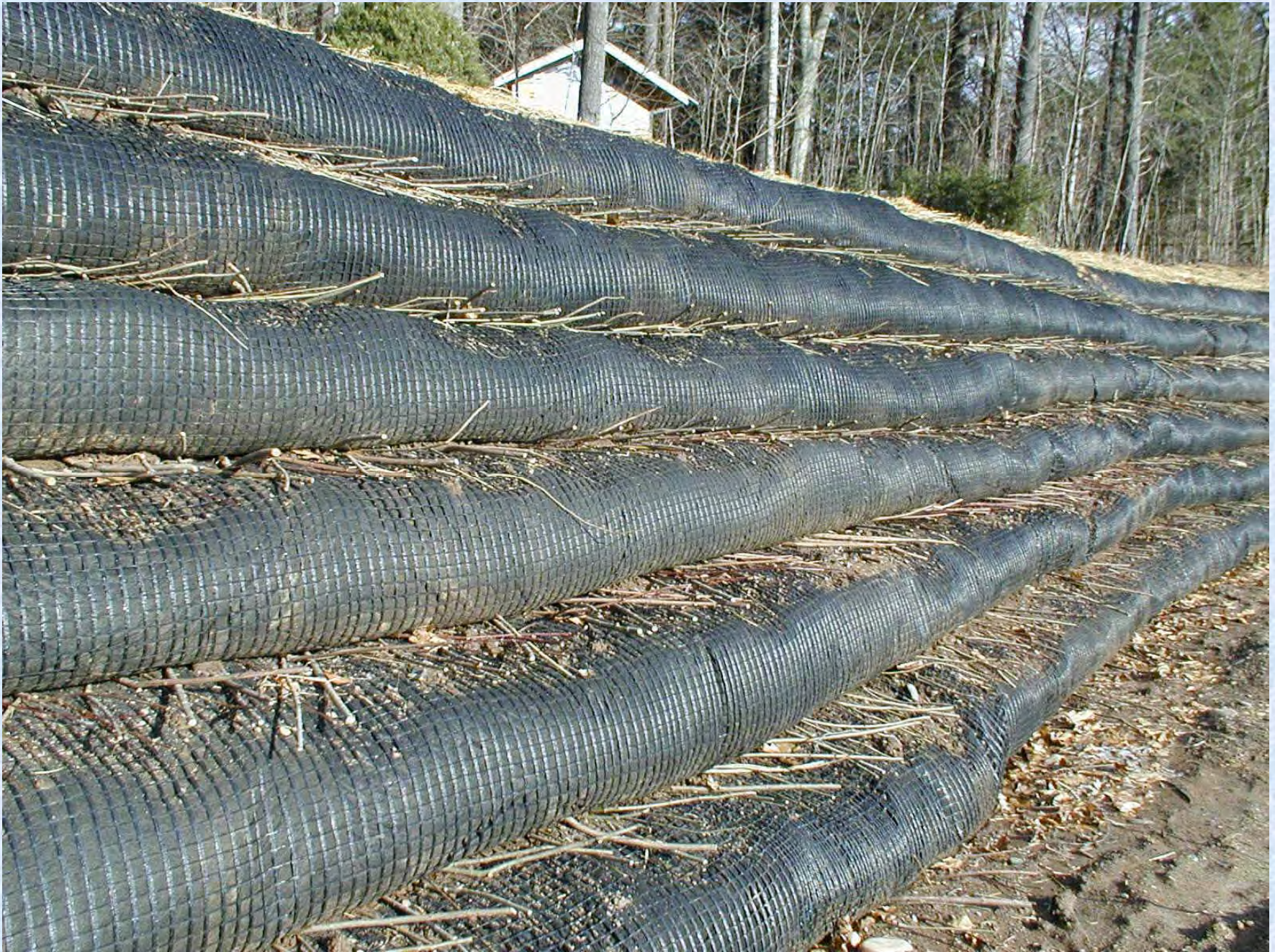
Vegetated Reinforced Soil Slope
