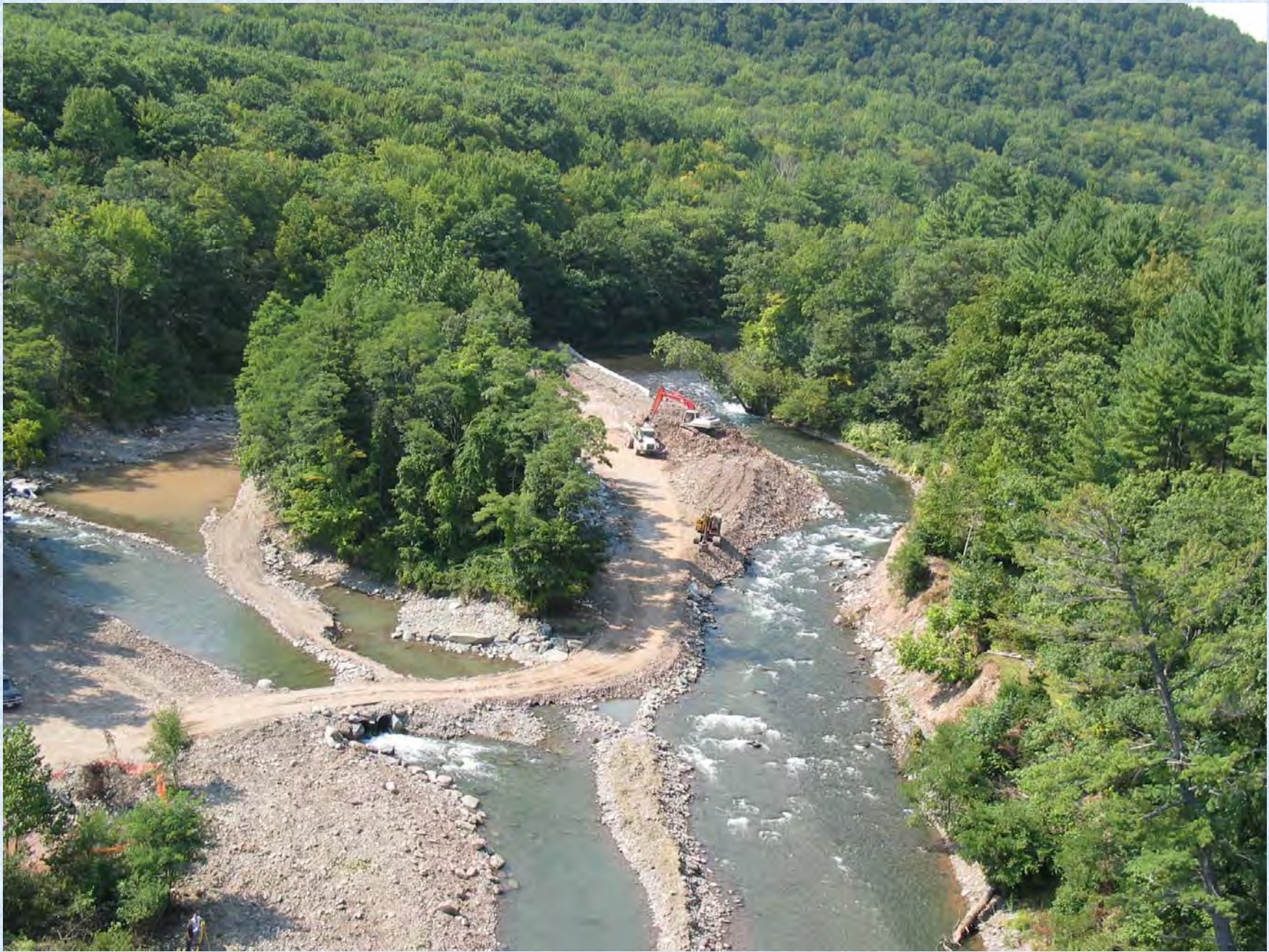
Project construction dewatering
