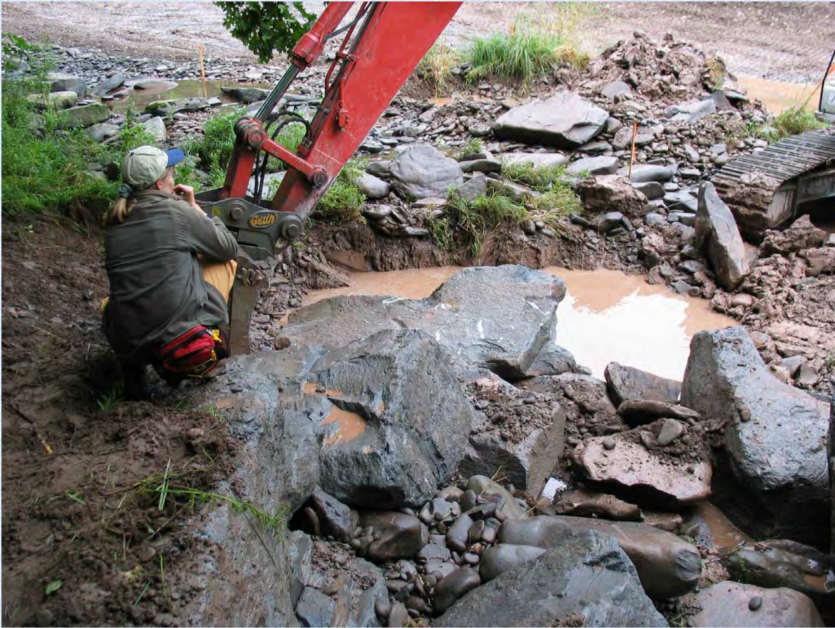
Constructing US boulder weir in glacial lake clay substrate
