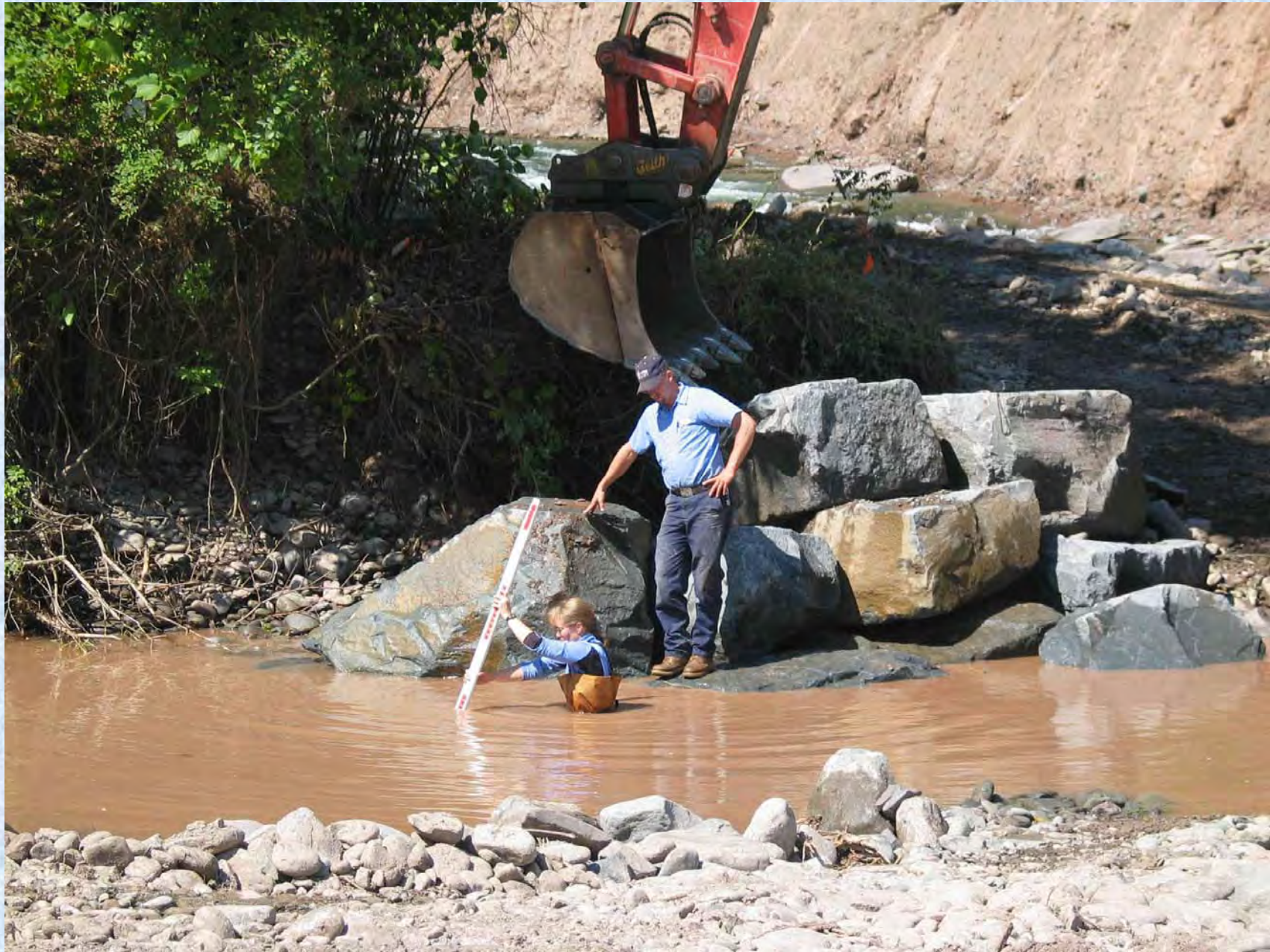
Constructing DS boulder weir in Esopus yooahoo
