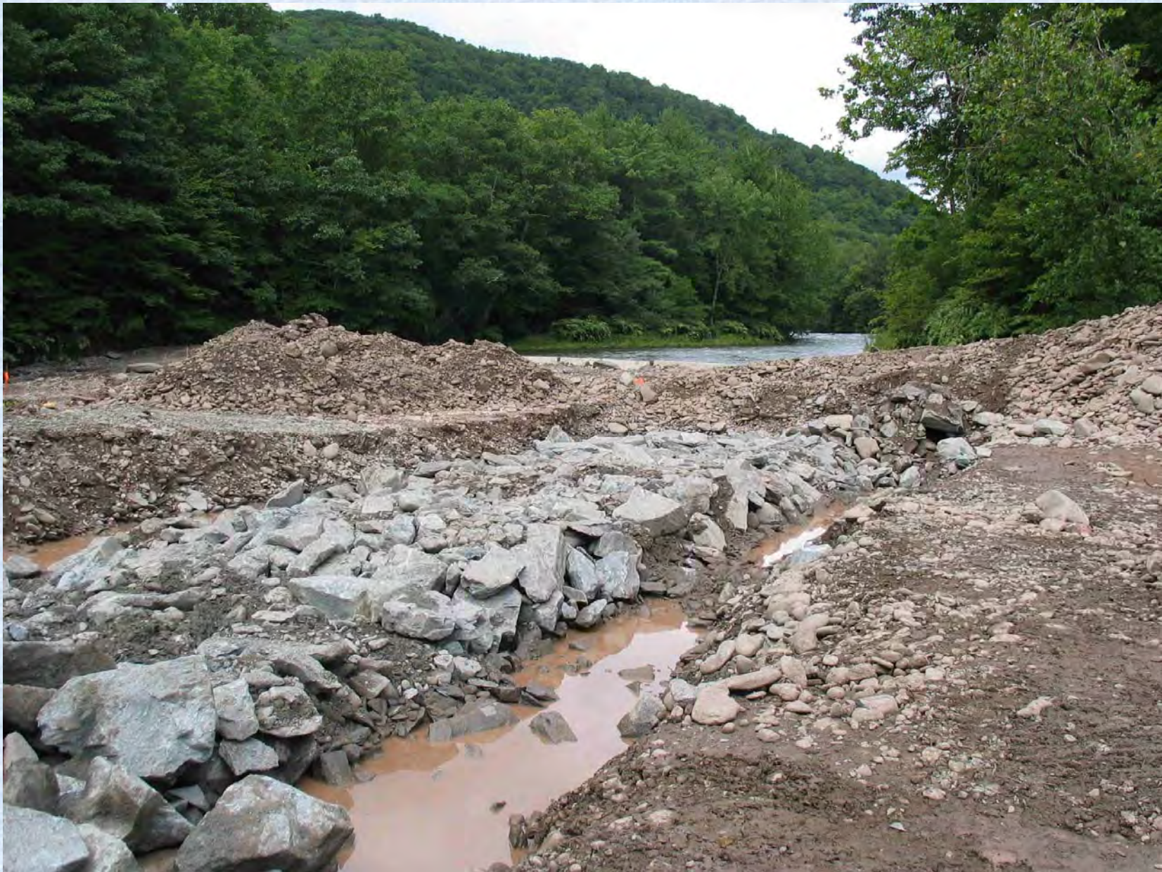
Installing channel blocks (buried rip rap) in flood plain
