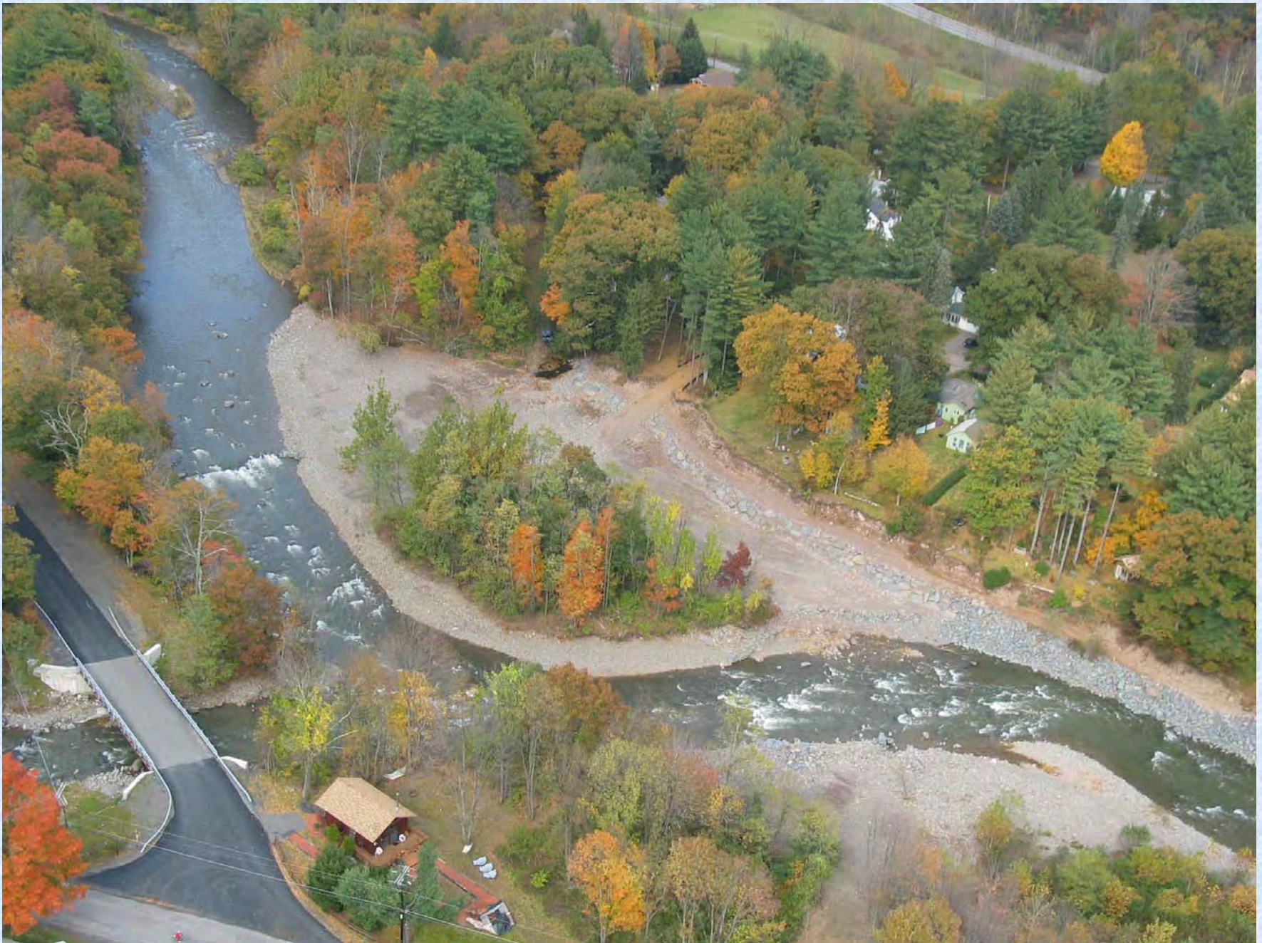
Completed channel work
