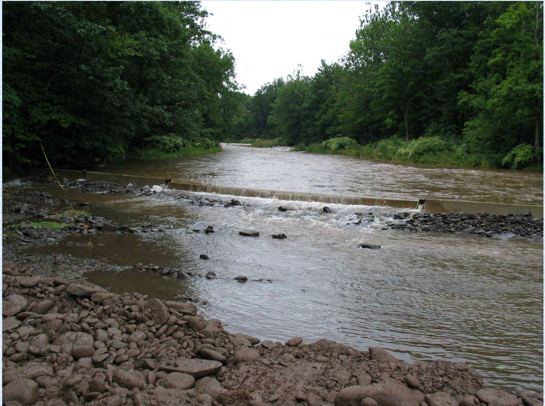
Diverting Esopus Creek high water with jersey barriers and berms 09.02.03
