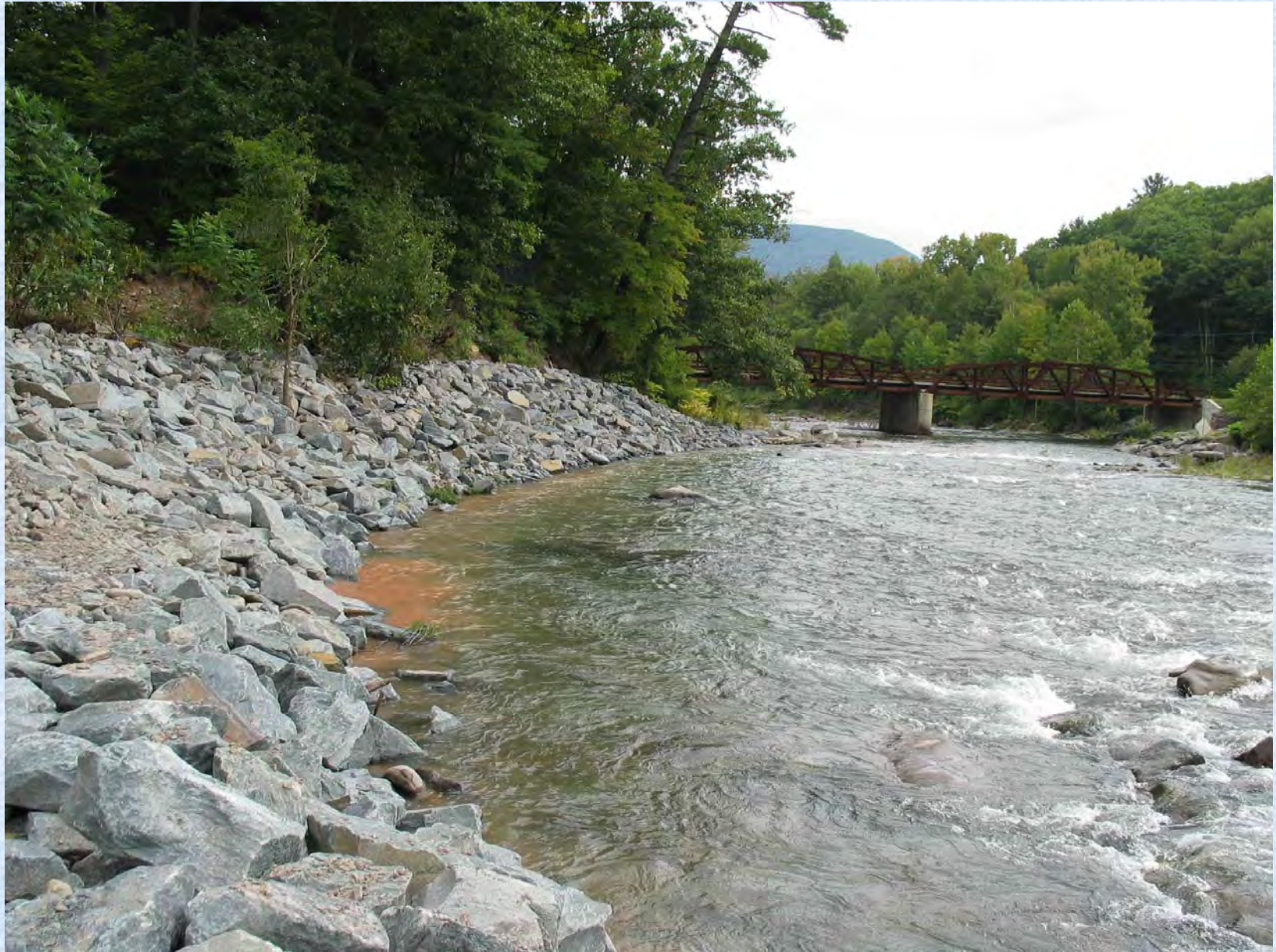
Stream bank armoring with graded rip rap
