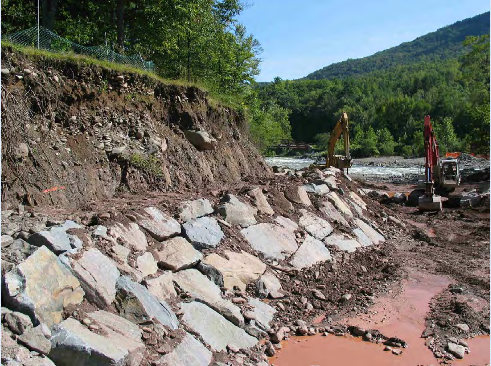
NRCS designed and installed “paved” rip rap
