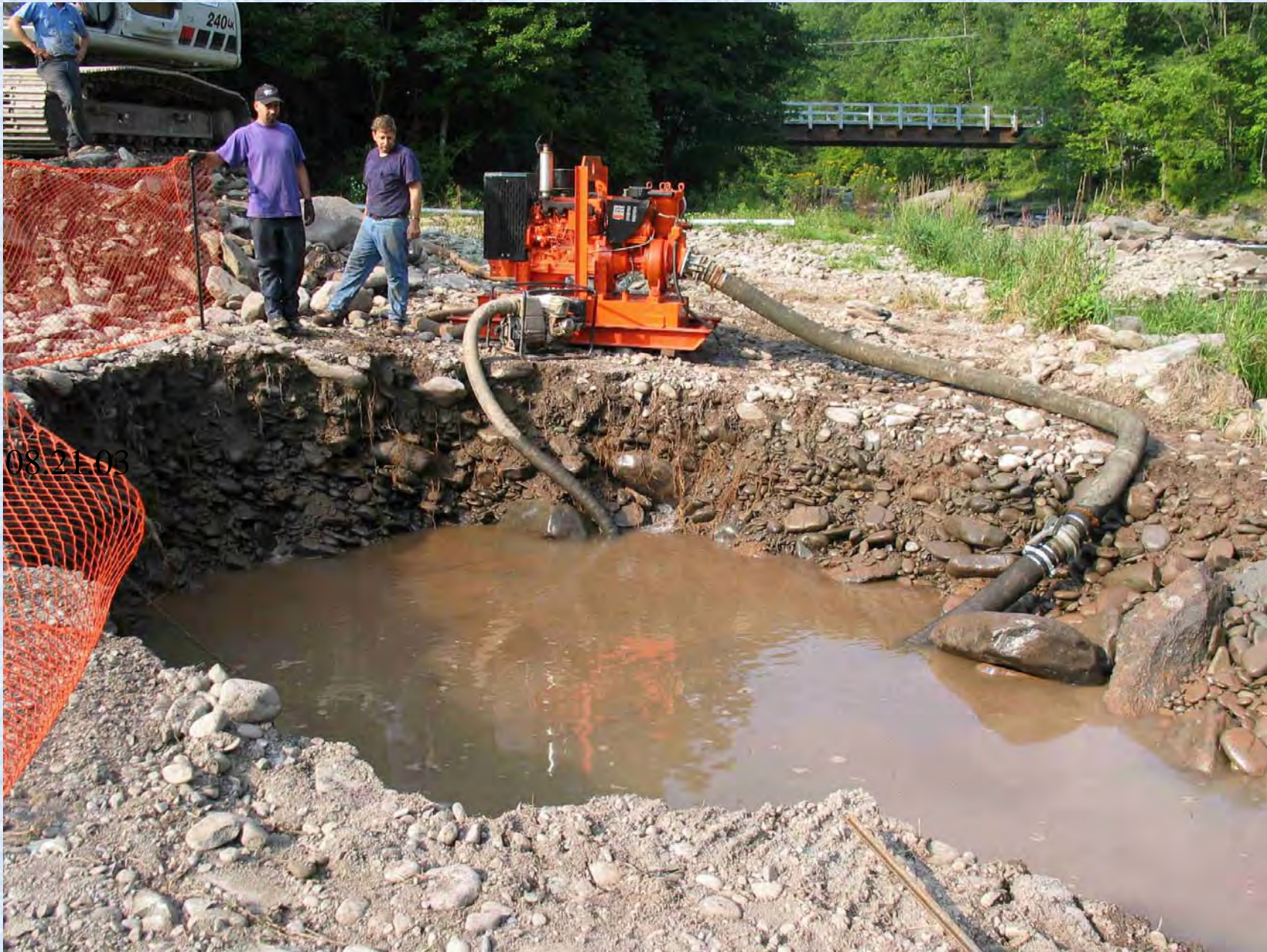
Dewatering in a saturated cobble bar
