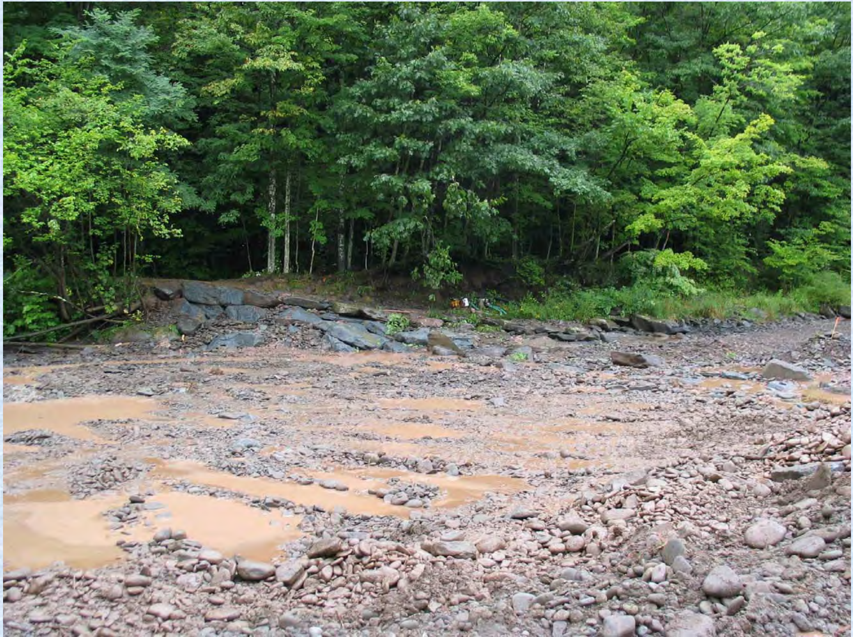
Completed US weir/vane
