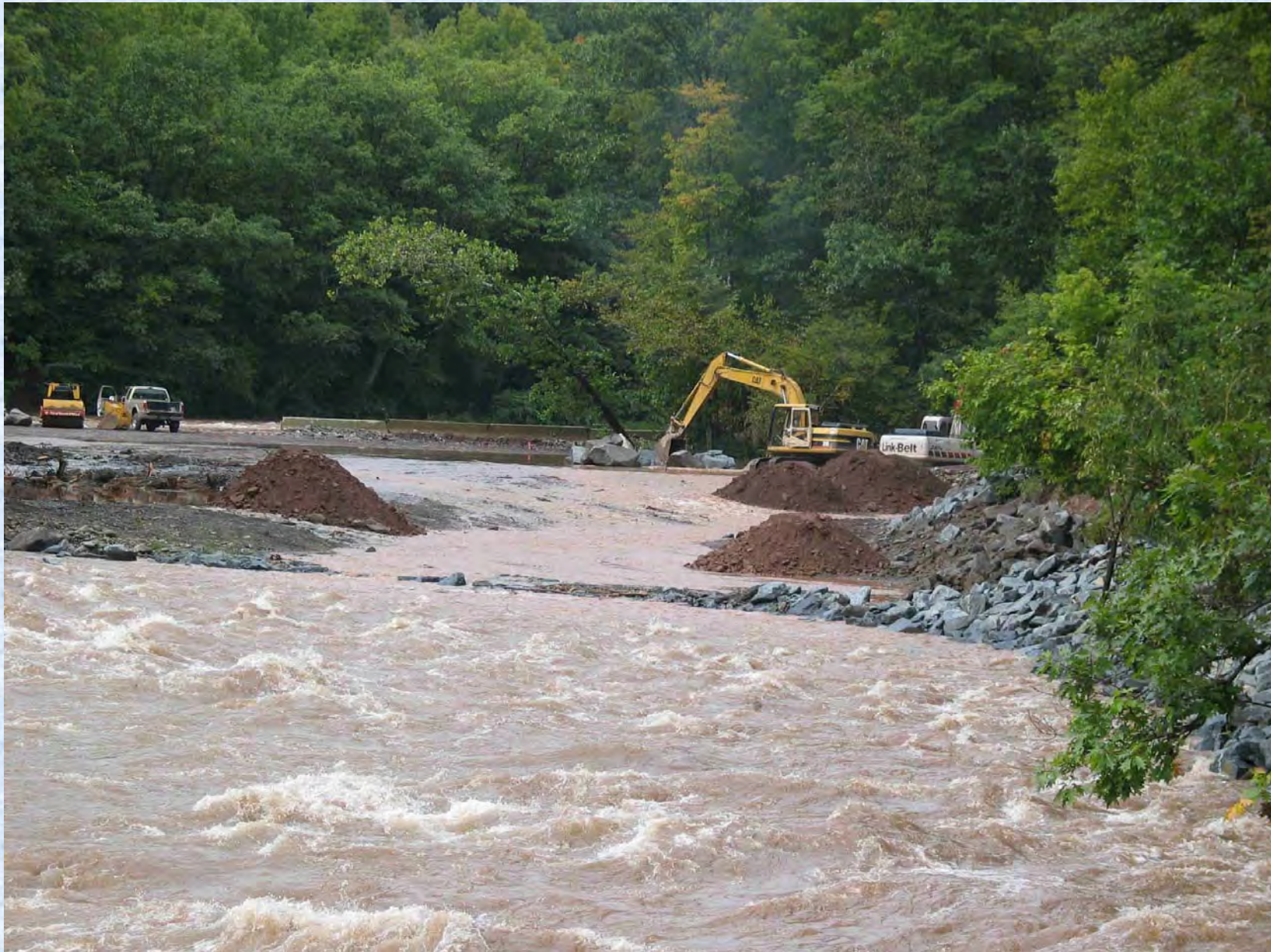
Flood flows over partially constructed floodplain
