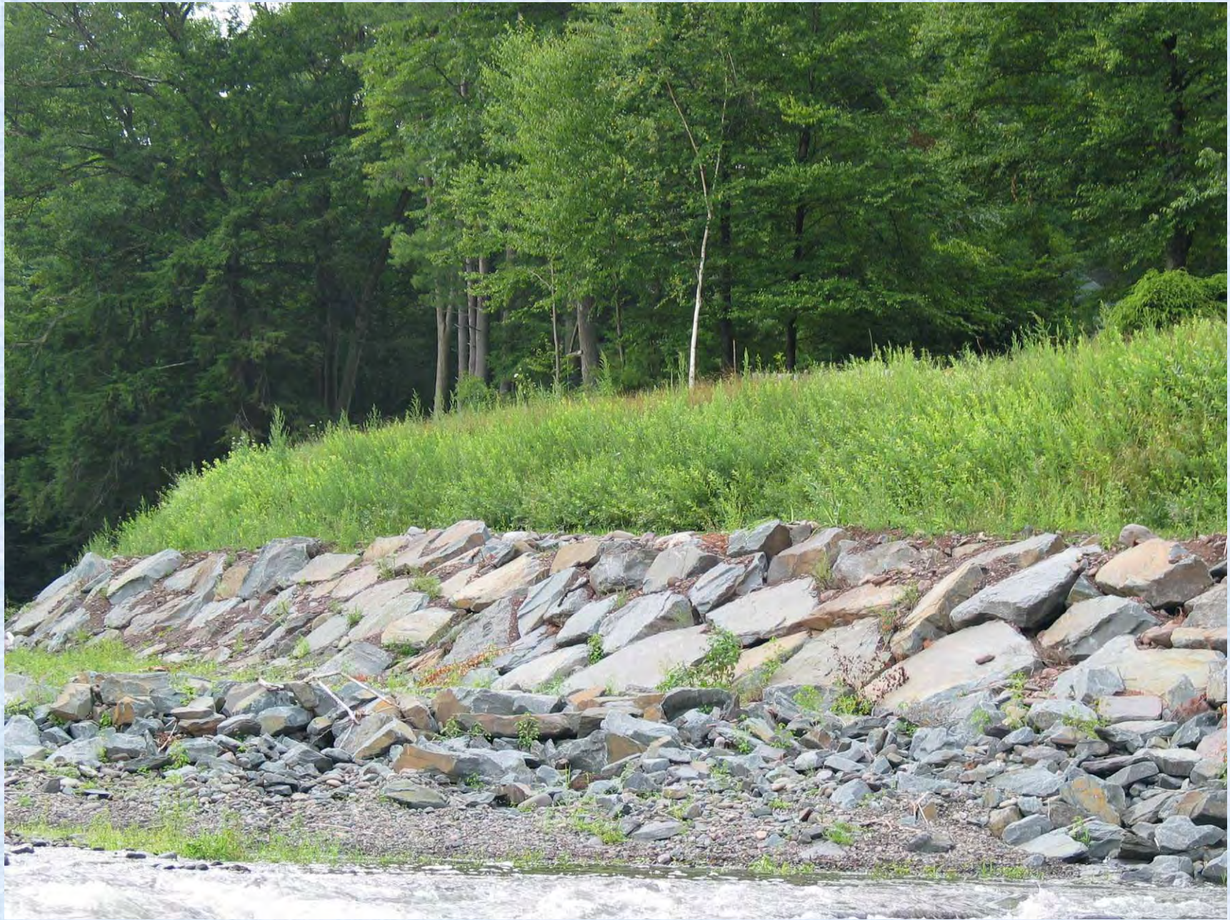
Vegetated Reinforced Soil Slope – first growing season
