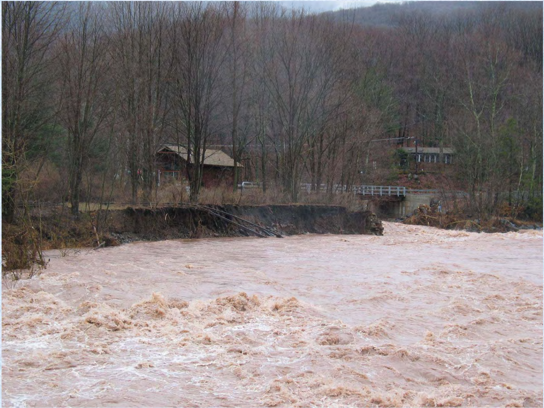
Stream bank and bed erosion
