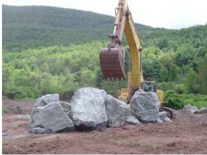
Rock being positioned for rock vane installation (left-above), rock vane designed to guide flow into bridge opening and ease pressure on the abutments and banks (center-above), and a fisherman seeking trout in the pool beneath a rock vane (right-above).
