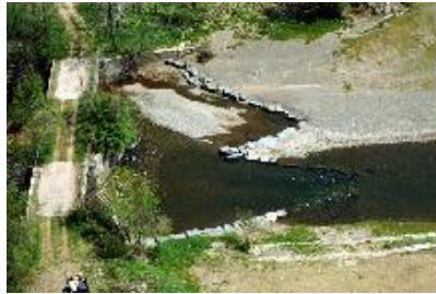
Rock being positioned for rock vane installation (left-above), rock vane designed to guide flow into bridge opening and ease pressure on the abutments and banks (center-above), and a fisherman seeking trout in the pool beneath a rock vane (right-above).
