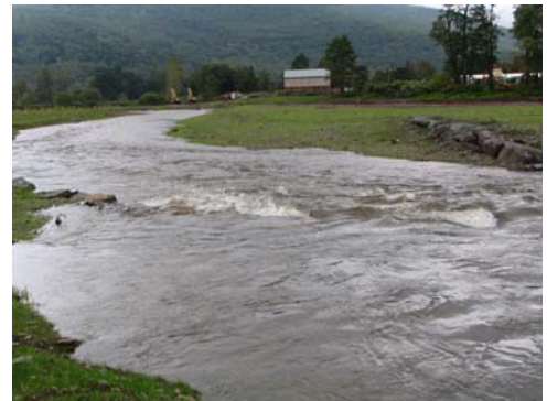
Laying the keyway back into the bank for a rock vane (left-above), rock vane designed to reestablish a riffle-pool sequence in a headwater stream (center-above), and high water moving over a vane, with the primary flow being moved to the center of the stream, reducing pressure on the banks (right-above).
