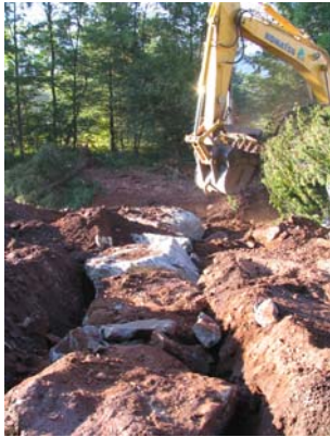
Laying the keyway back into the bank for a rock vane (left-above), rock vane designed to reestablish a riffle-pool sequence in a headwater stream (center-above), and high water moving over a vane, with the primary flow being moved to the center of the stream, reducing pressure on the banks (right-above).
