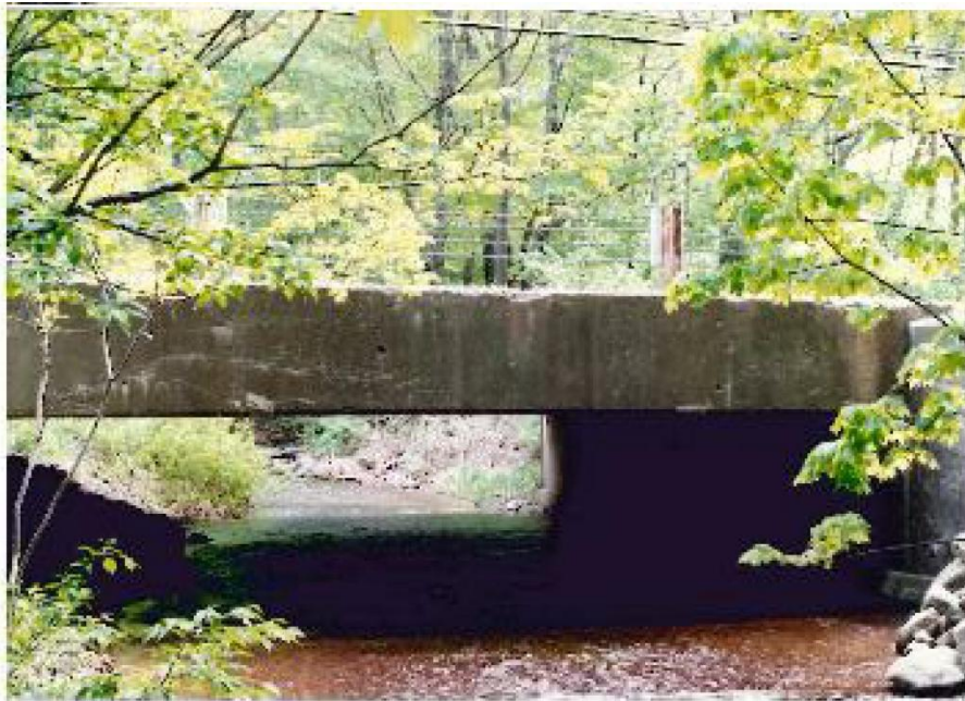
Historic Photo of Culvert Circa 1990
