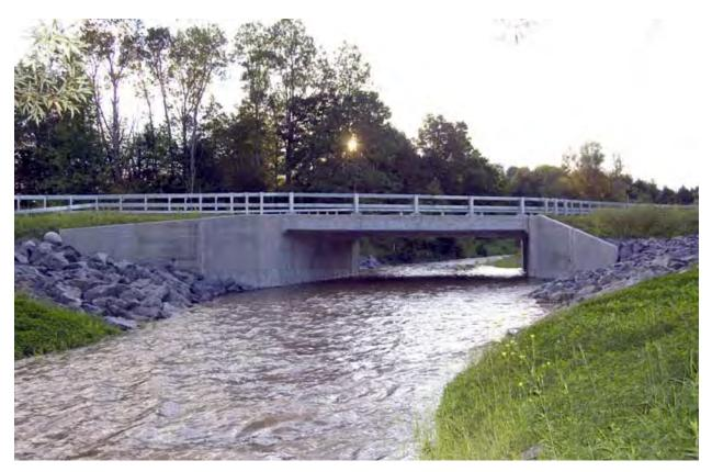
Figure 4-2: Example Precast Culvert (over a stream, not a floodplain) Source: Binghamton Precast & Supply Corp
