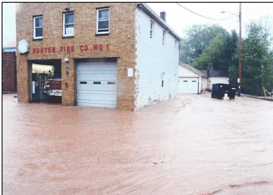
Figure 3-5 Floodwaters at Hunter Firehouse Tropical Storm Irene, August 28, 2011
