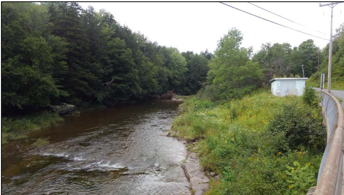
Figure 4-8 Dam Located Downstream of Elka Park Road Bridge
