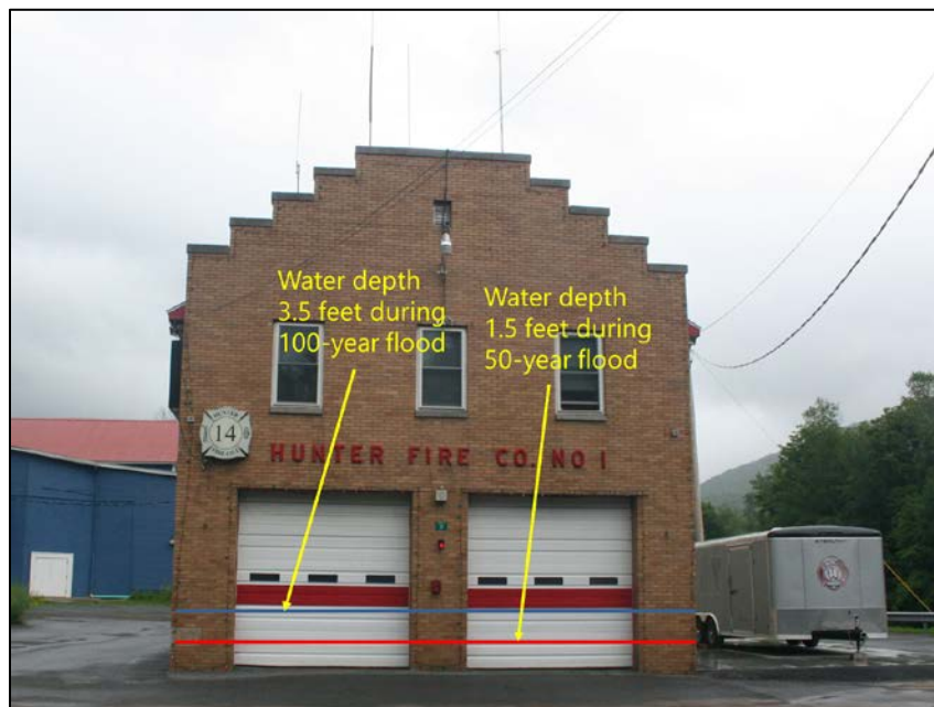
Figure 4-1 50- and 100-Year Flooding Depths Hunter Fire Station on Bridge Street
