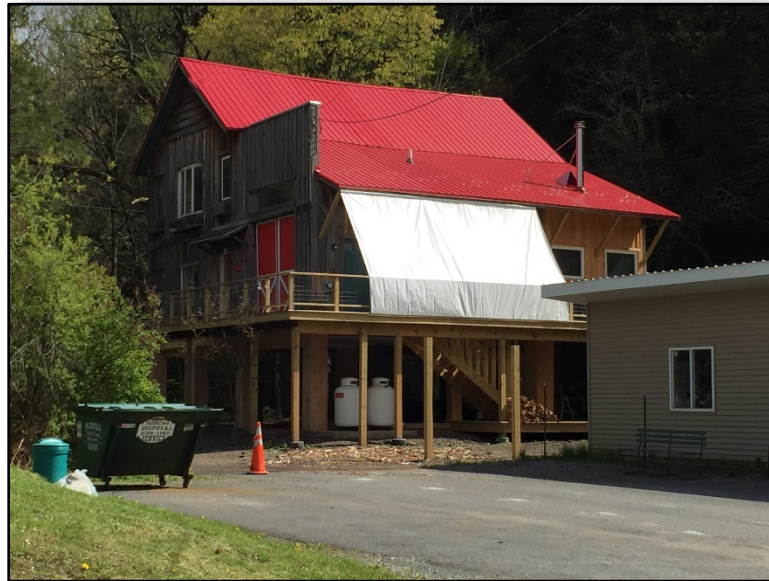
Figure 6-4 Example of an Elevated Structure
