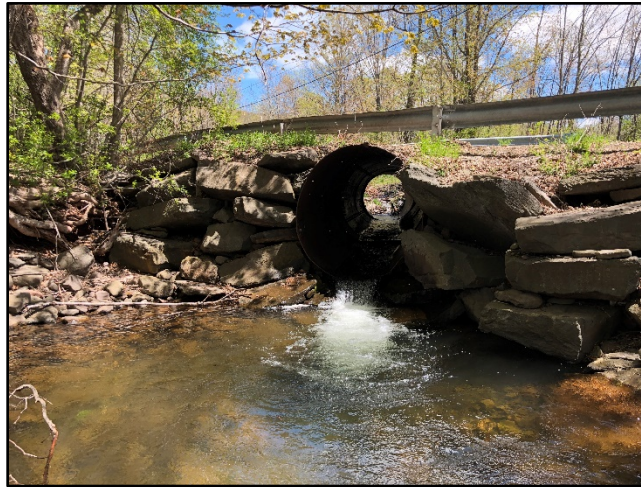
Figure 4-47 Glen Avenue Culvert over Mad Brook
