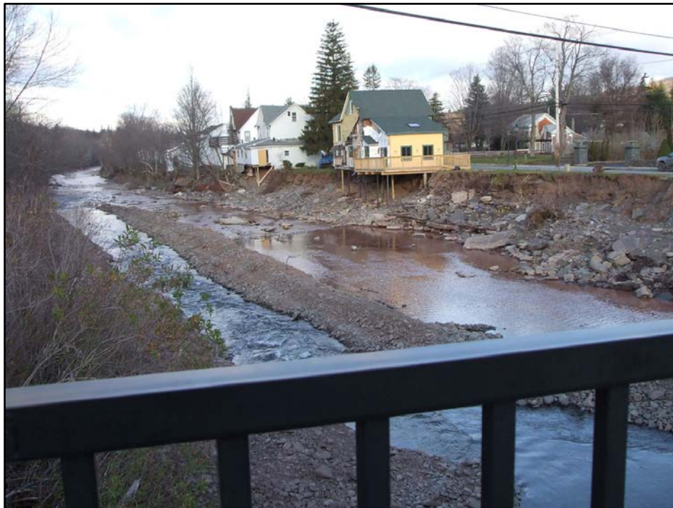
Figure 3-7 Homes along Schoharie Creek following Tropical Storm Irene, August 28, 2011
