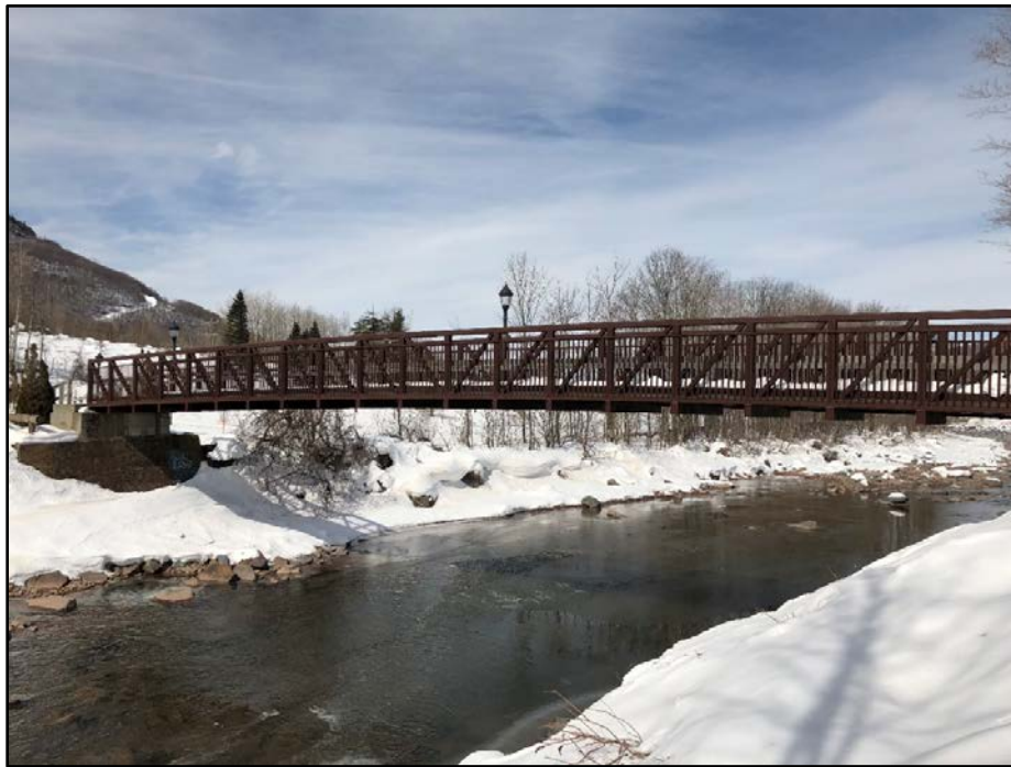
Figure 4-10 Pedestrian Bridge over Schoharie Creek
