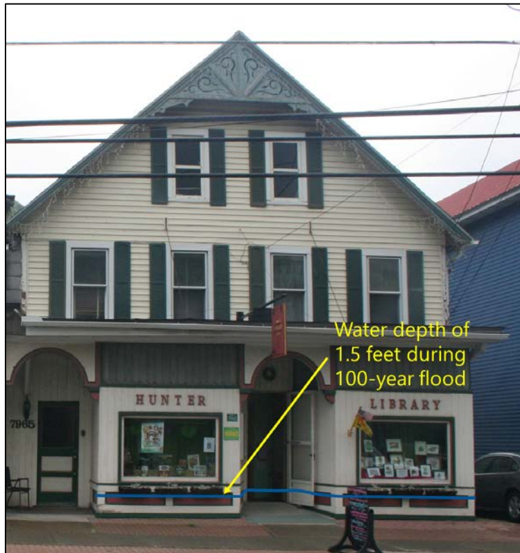
Figure 4-4 100-Year Flooding Depth Hunter Library on Main Street
