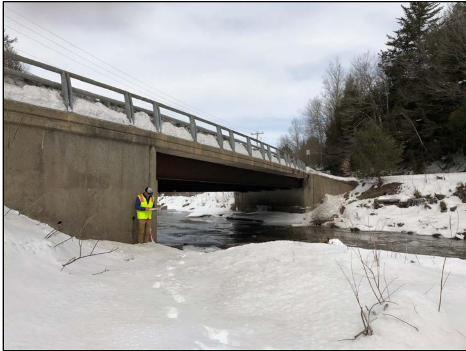
Figure 4-7 Elka Park Road Bridge over Schoharie Creek
