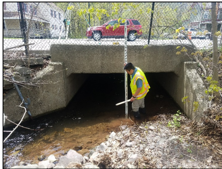
Figure 4-46 Main Street Culvert over Mad Brook
