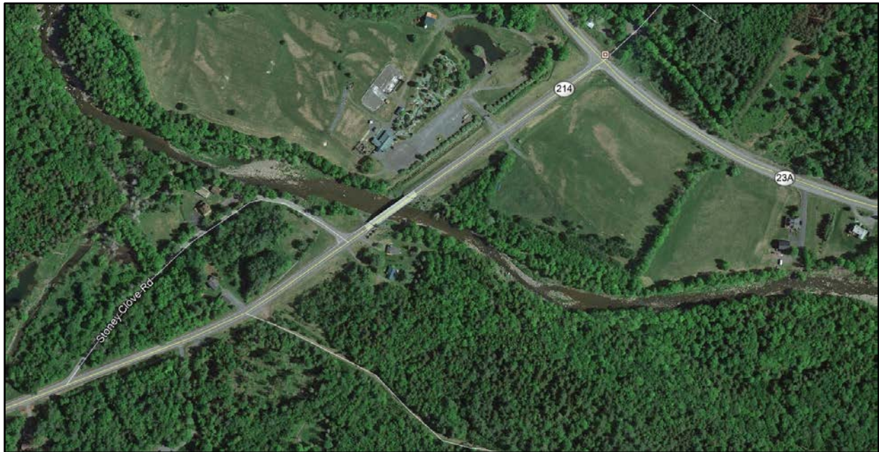
Figure 4-9 NYS Route 214 Bridge over Schoharie Creek
