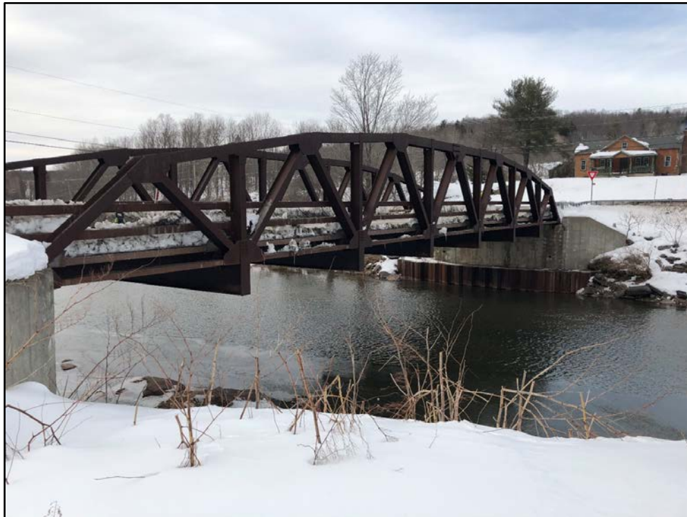
Figure 4-29 Deming Road over Schoharie Creek
