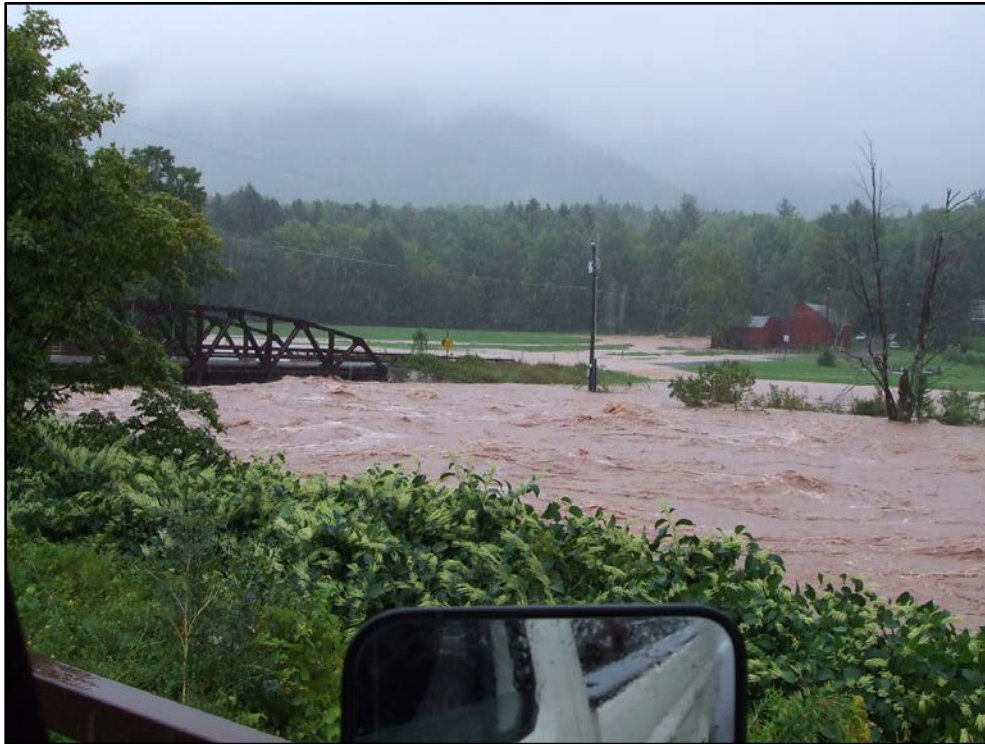
Figure 4-30 Deming Road over Schoharie Creek during Tropical Storm Irene
