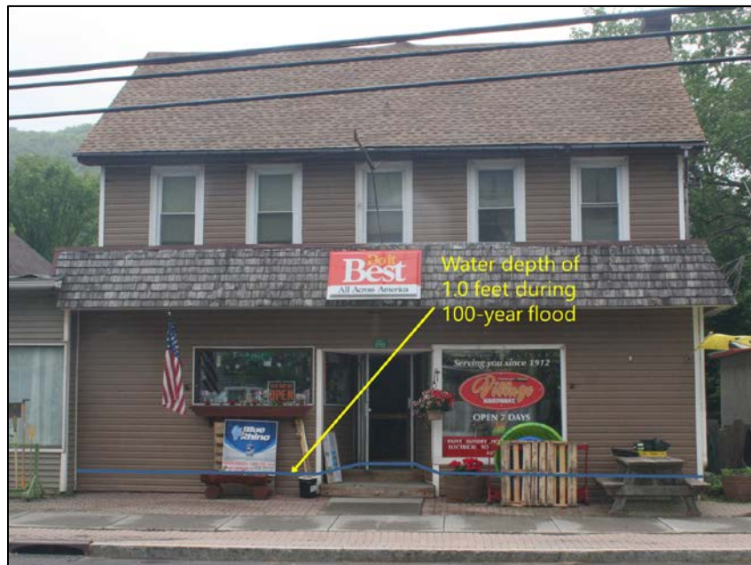
Figure 4-5 100-Year Flooding Depth Hardware Store on Main Street
