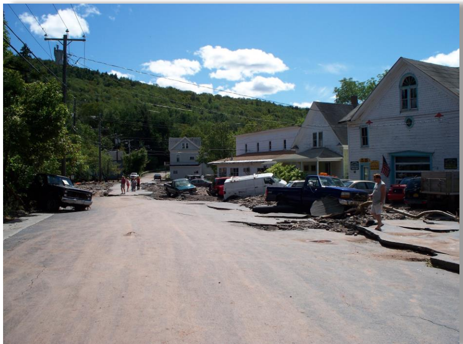
Figure 3-6 View of Railroad Avenue and Legg's Garage the day after the flood
