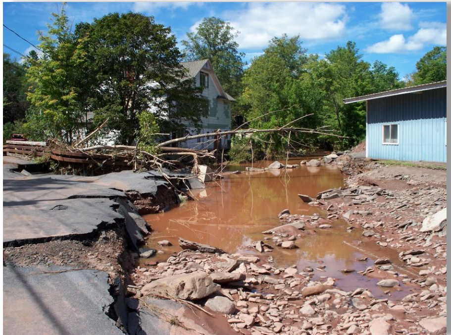
Figure 4-26 Tannersville Highway Department Garage following Tropical Storm Irene
