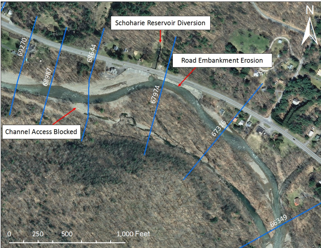
Figure 4-38 Post-Irene Channel Conditions in the Vicinity of the Shandaken Tunnel
