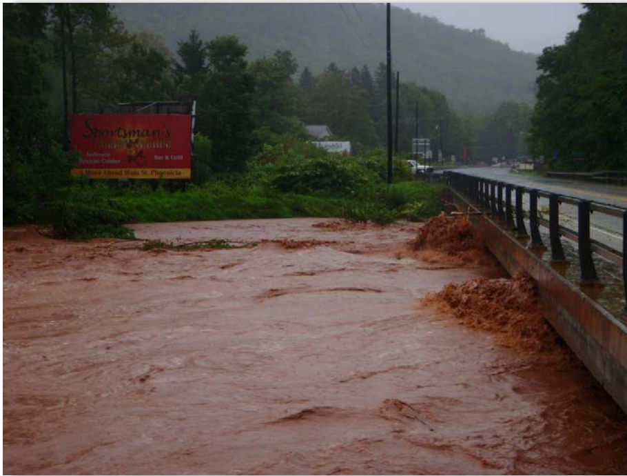
Figure 3-4 Esopus Creek Nearly Reaching Deck of State Route 28 Bridge in Shandaken
