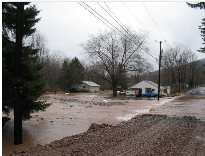
Figure 3-2 Fox Hollow Road Washed Out During the 2005 Flood Event
