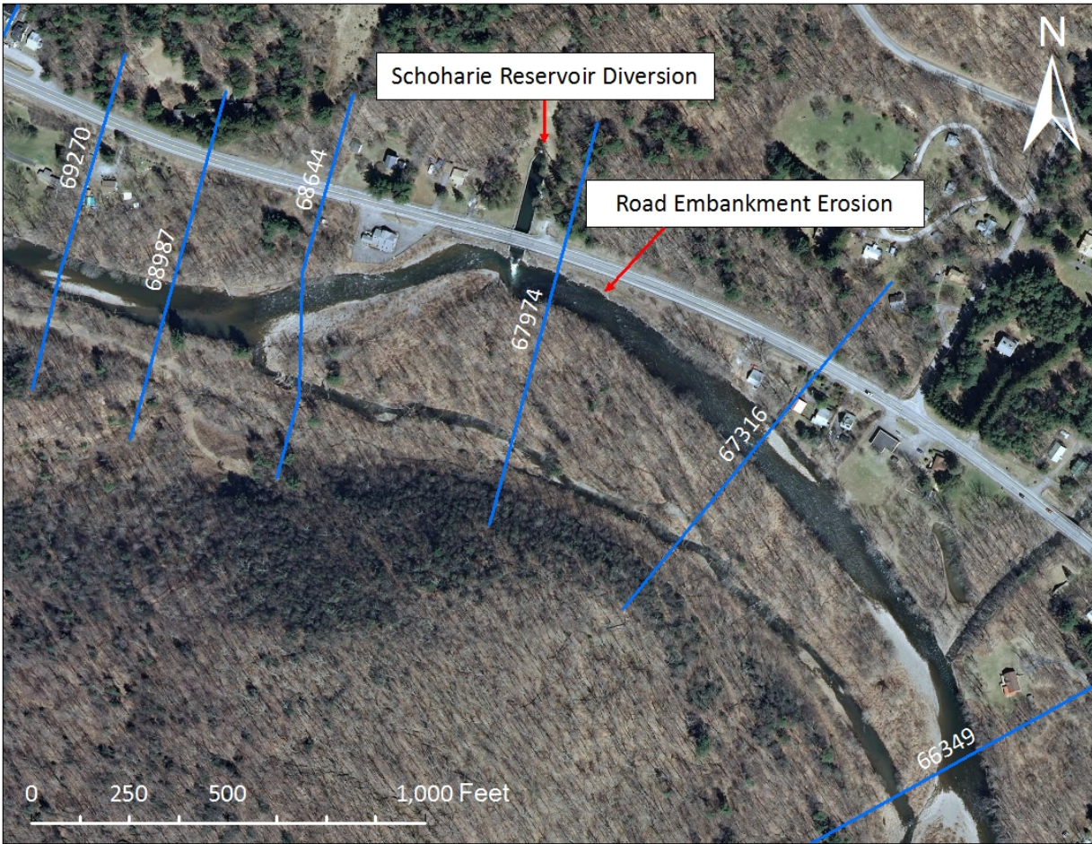
Figure 4-37 Pre-Irene Channel Conditions in the Vicinity of the Shandaken Tunnel
