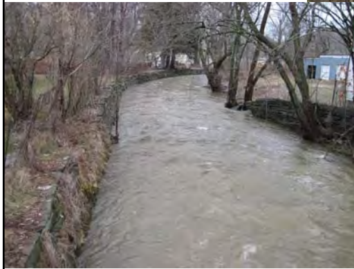
Mead Street Bridge and Downstream Channel
