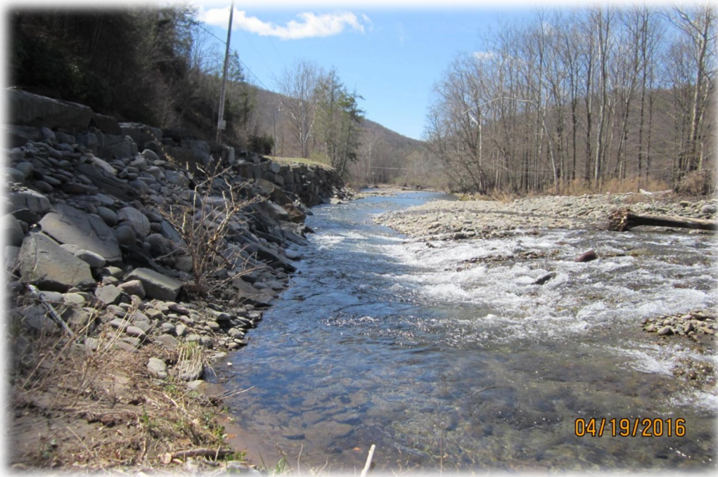
Rondout Creek flows against the stone wall supporting Peekamoose Road (Photo 1)
