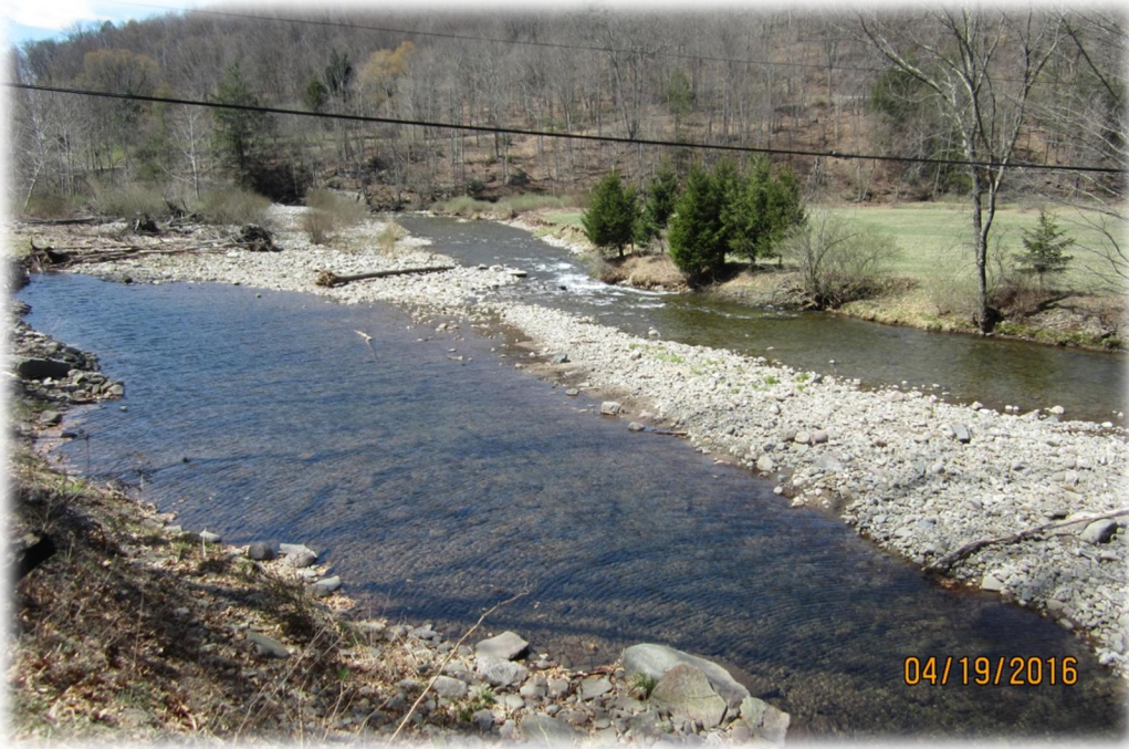
Rondout Creek Channel splits creating erosion of left and right banks. (Photo 3)
