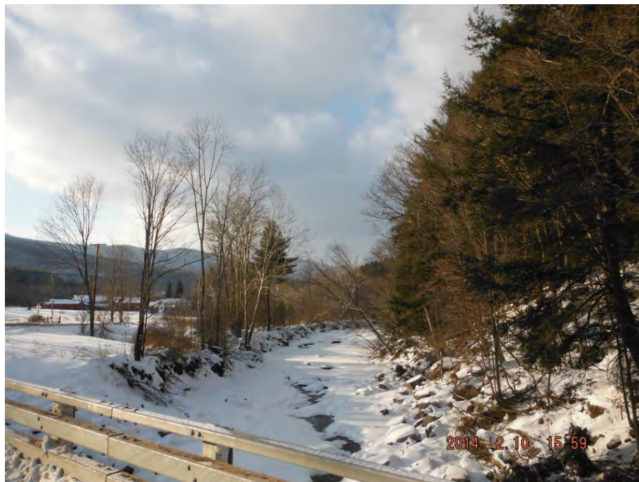
West Kill viewed from Route 6 bridge
