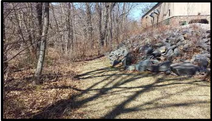
**Figure 17: Looking Upstream at Rip Rap Embankment at Waste Water Treatment Plant (Building B11)**
