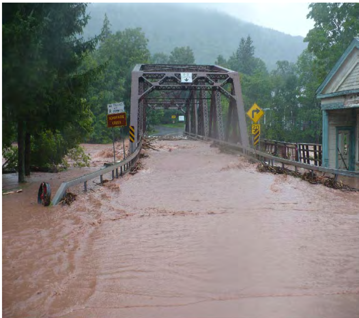
Figure 1.—Bridge over Schoharie Creek near Lexington, N.Y., Aug. 28, 2011. Photo taken by Travis L. Smith (USGS Troy NYWSC).
