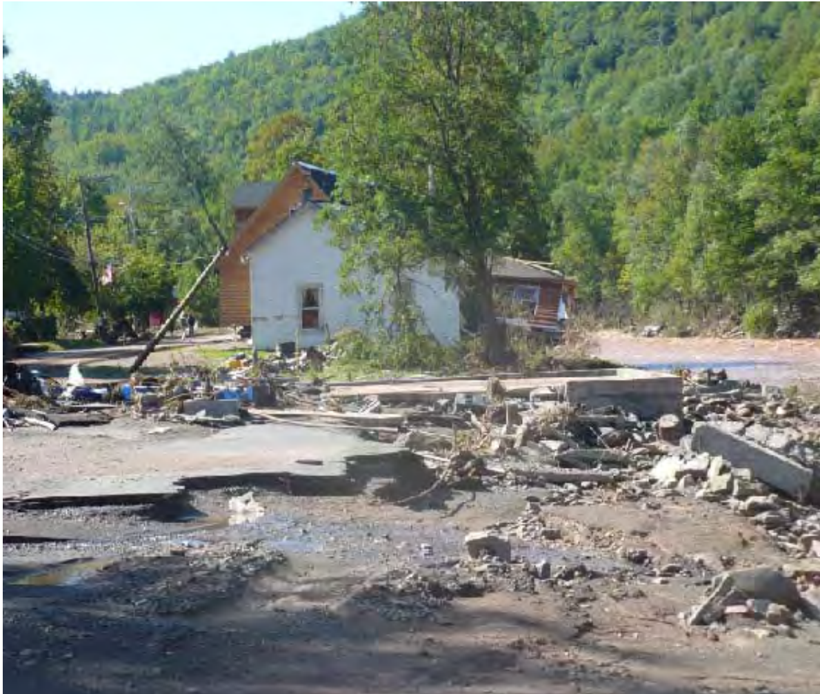
Figure 3.-- Road and homes damaged along the Schoharie Creek near Prattsville, NY, Aug. 29, 2011. Photo taken by K.D. Reisig (USGS Troy NYWSC).
