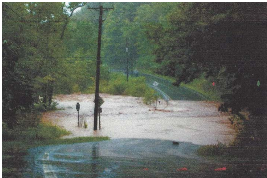
Figure 2-6 Project Area 1: Floodwater from the Manor Kill flooding intersection of Pangman Road and Route 990V during Tropical Storm Irene, August 2011.
