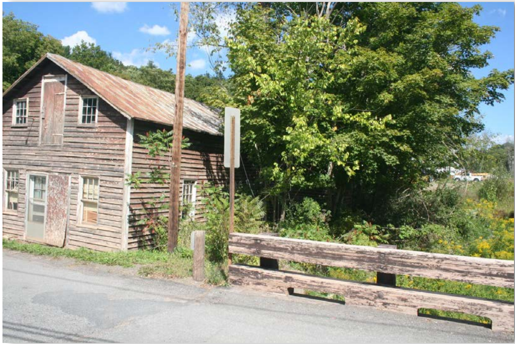
Figure 2-13 Study Area 3: Durham Road Bridge and Abandoned Structure
