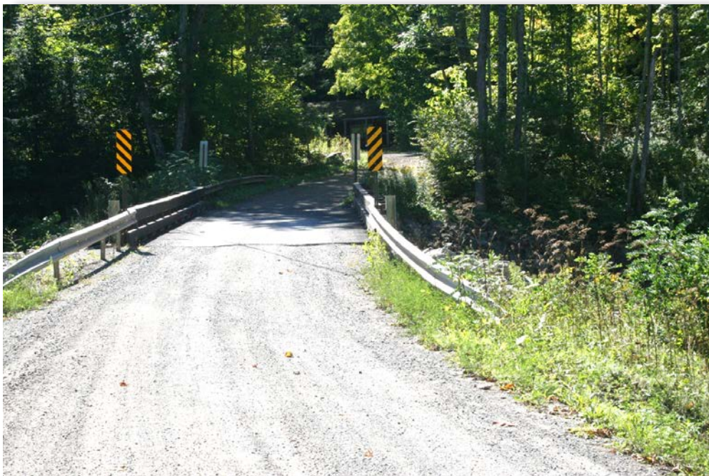
Figure 2-4 Project Area 1: Pangman Road Bridge
