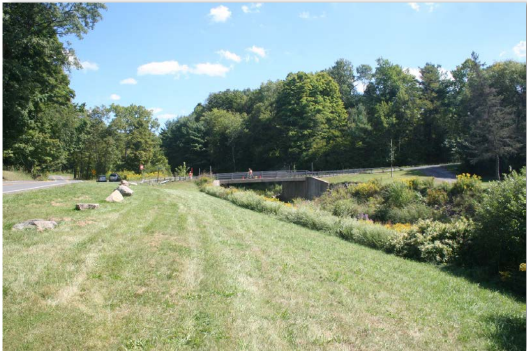
Figure 2-10 Study Area 2: View of South Mountain Road Bridge from downstream
