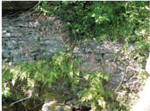
Stone gabion revetment on right bank (P7190130)
