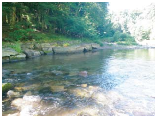
Placed quarry rock forming grade control (P7290125)
