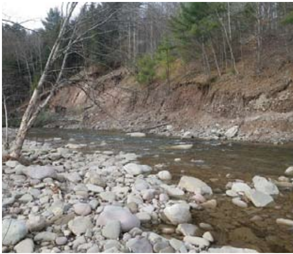
Slope failure on the right bank across from cobble point bar. (IMG1744)
