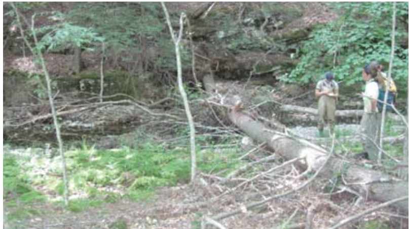
Large obstructions in side channel (B332)
