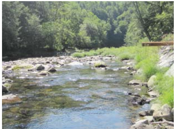
Piped outfall conveying flow from Frost Valley Road (A263)
