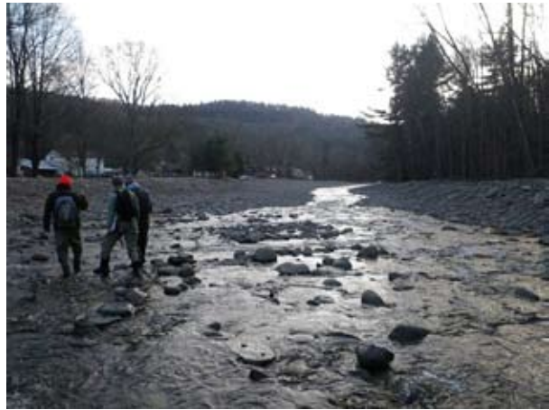
Appropriately sized main channel. Flow is diverted by a berm upstream. (IMGP1769)
