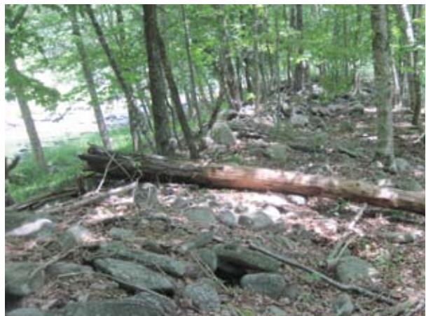
Berm along left bank (B288)
