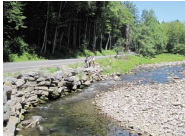
Stacked rock revetment protecting Frost Valley Road (A280)
