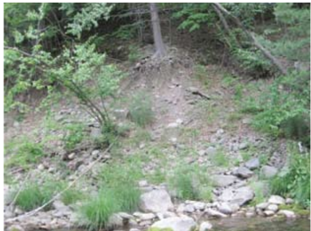
Stabilizing slope failure on right bank (A334)
