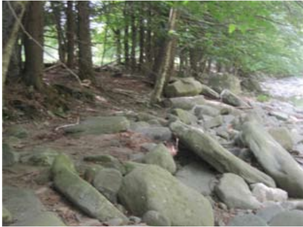
Boulder revetment along left bank (B293)
