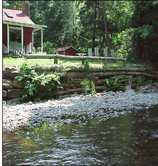
Figure 4 Mowing to the edge of the stream leads to bank failure. This bank has been reinforced with log cribbing.
