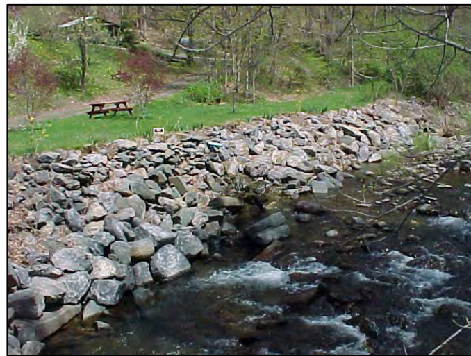
Figure 10 Joint plantings at this site would increase stream bank stabilization and improve fish habitat
