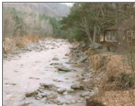
Figure 3 Erosion from 1996 Flood at VanNorstrand Property, looking upstream
