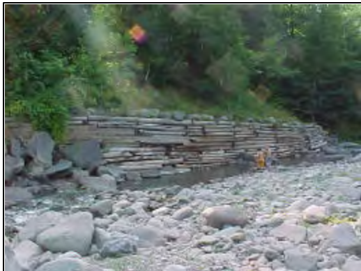
Figure 10 Log cribbing August 16, 2001
