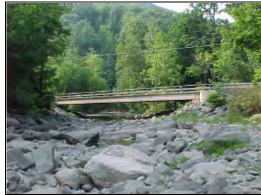
Figure 11 NYS Route 214 bridge
