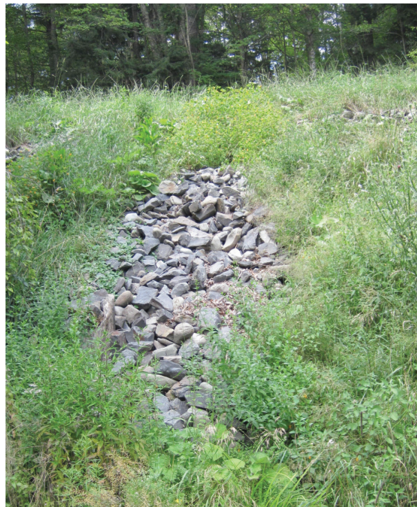
Rip-rap revetment protecting Frost Valley Road (A183)
