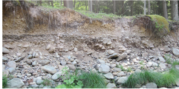
Active hydraulic erosion with soil failure site (A175)
