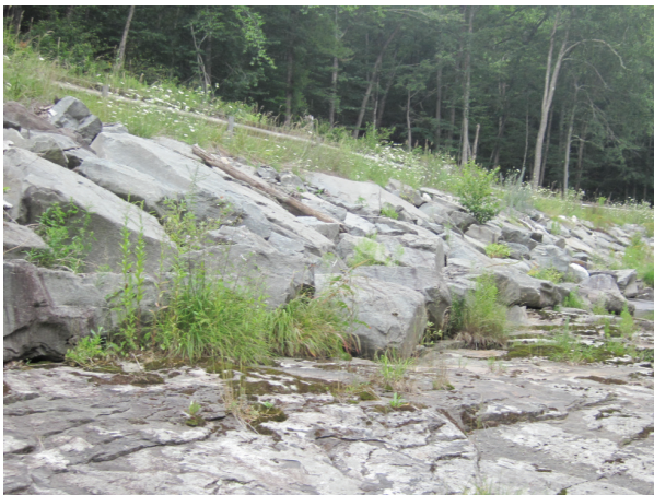
Sloped stone revetment on right bank (A208)
