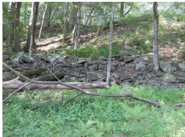
Stone berm along right bank (A218)
