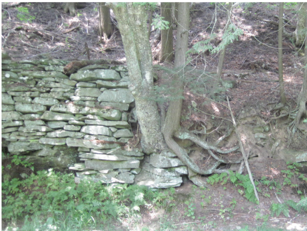
Stacked rock berm in right floodplain (A181)
