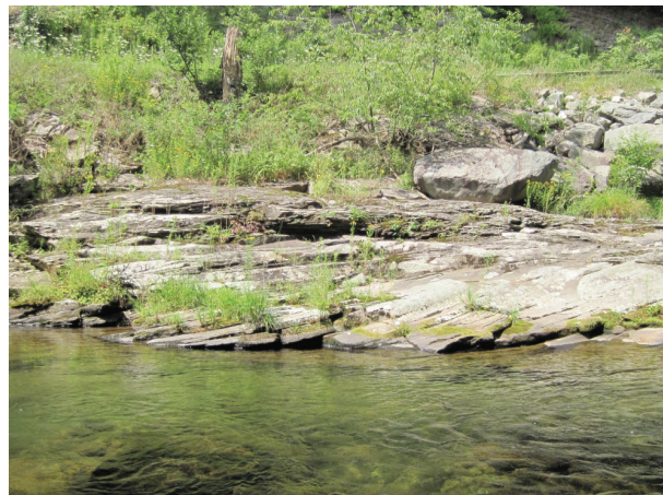
Revetment keyed into exposed bedrock (A211)
