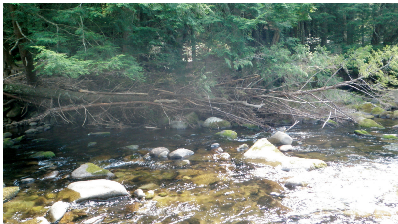
Downed tree causing bank scour (P7280110)
