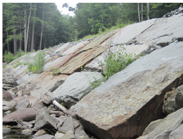
Sloped stone and rip-rap revetment (A188)
