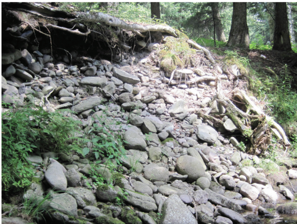
Eroding segment on right bank (A146)
