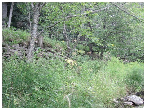
Dumped cobble revetment on right bank (A202)
