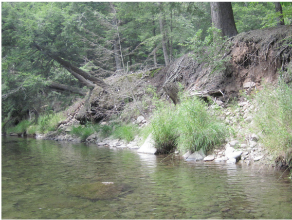
Eroding right bank (A159)
