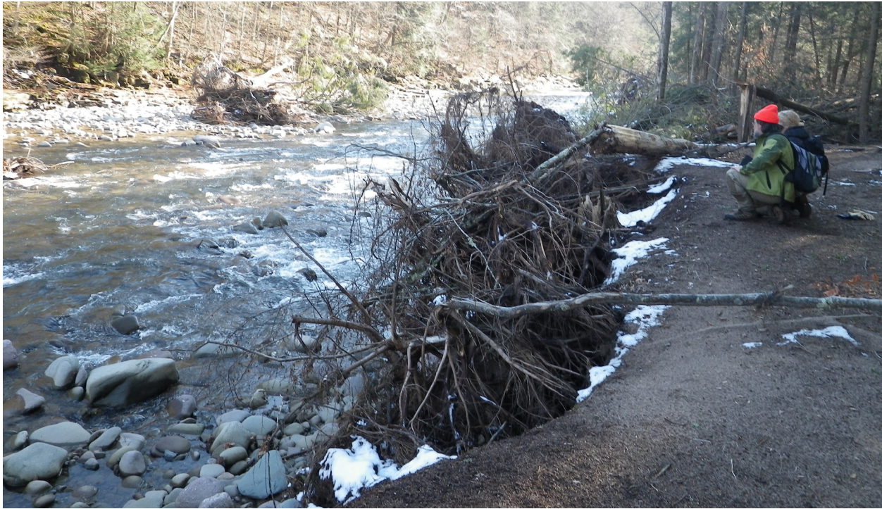
Significant erosion of the right bank, with mature trees undercut. Here, at Station 5600, flow from the main channel accesses the floodplain during overbank flow events, concentrating in a back-channel running nearly the length of this MU2. (2267)
