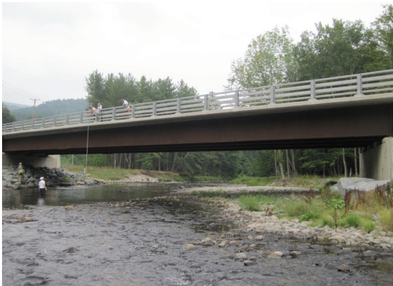
Frost Valley Road bridge (A11)
