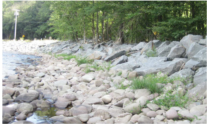
Right bank revetment (A345)
