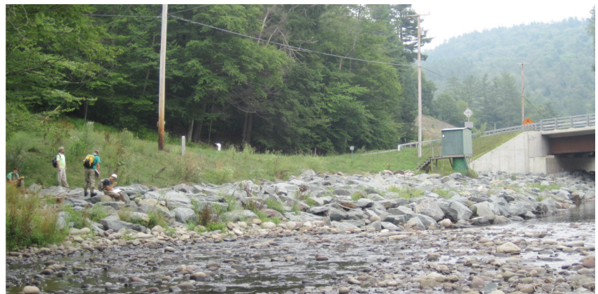
Left bank revetment (B355)
