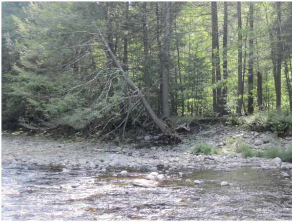
Eroding segment on right bank (A339)
