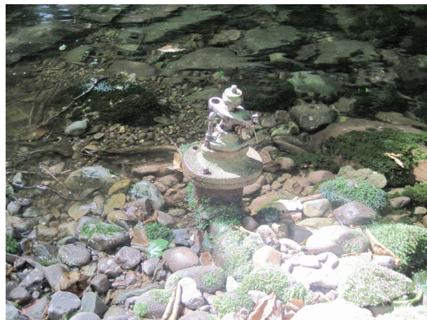
Piping in channel bed (A456)
