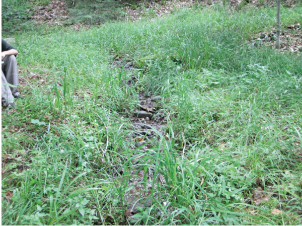
Chute conveying intermittent seepage (A825)
