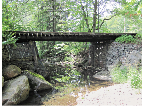
Private bridge (A775)
