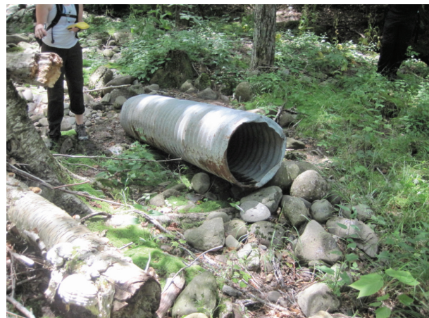
Culvert and woody debris (A789)
