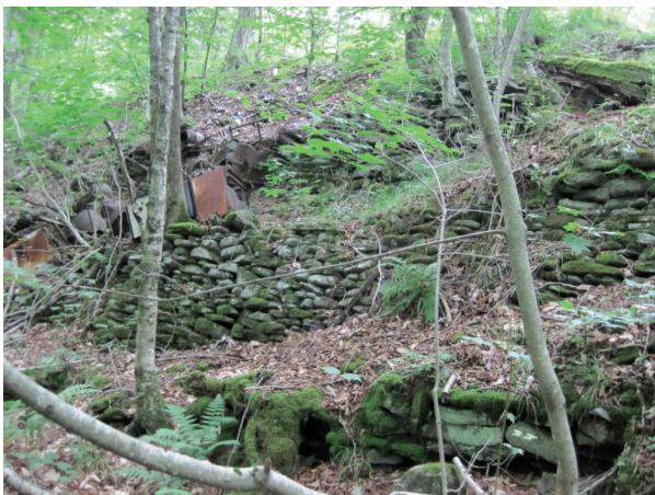
Three level stone wall terrace on right bank (A824)
