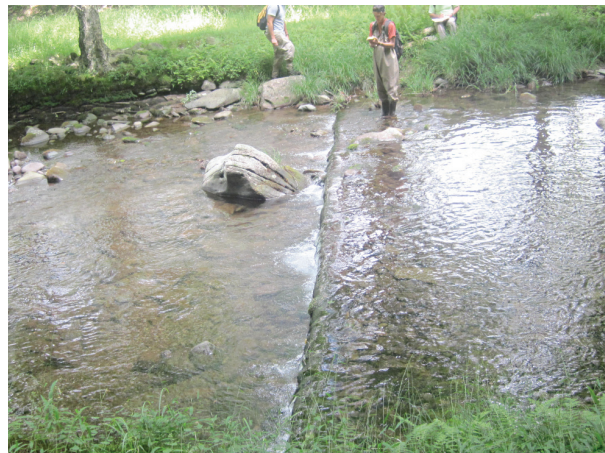
Log check dam and log cribbing (B912)
