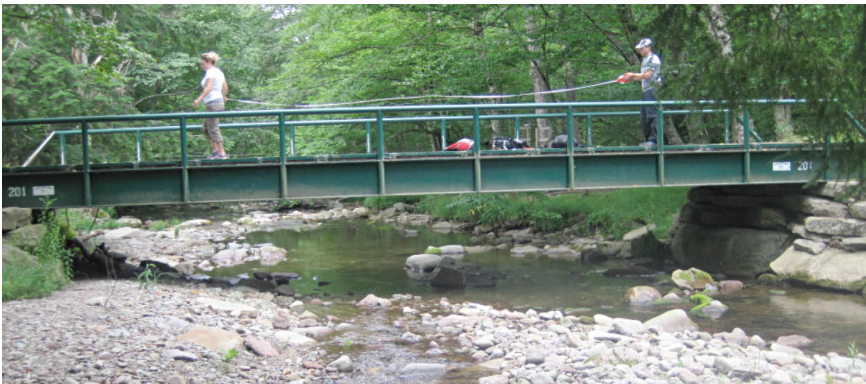
East Entrance Bridge (A1016)
