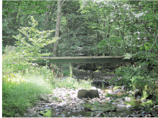
East Entrance Bridge (B893)
