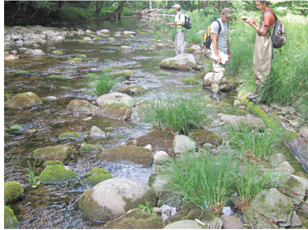
Log cribbing revetment on right bank (B909)
