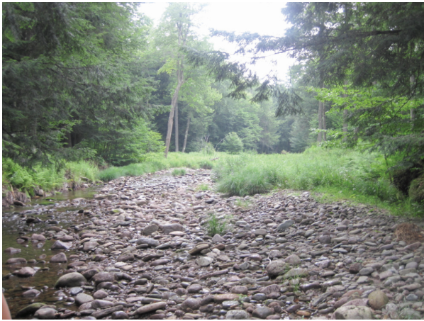
Center bar upstream of bridge (A1011)
