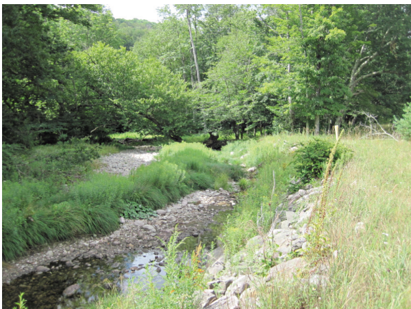
Sloped stone revetment on right bank (A1038)
