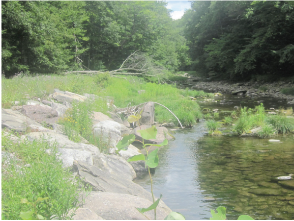
Sloped stone revetment stabilizing bank (B976)
