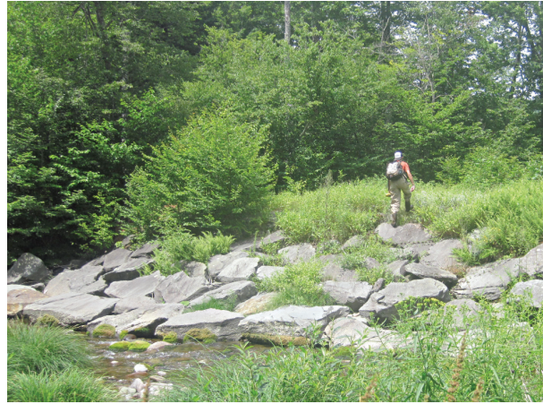
Sloped stone revetment (B959)
