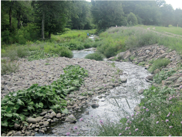
Rip rap revetment (B1021)
