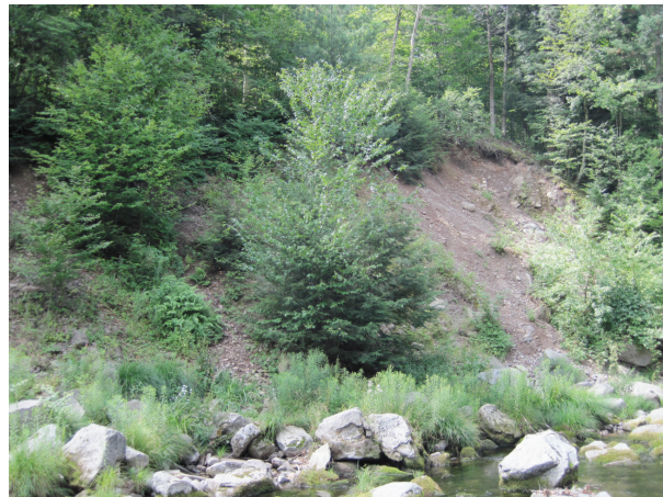
Re-vegetating hill slope failure (A1064)
