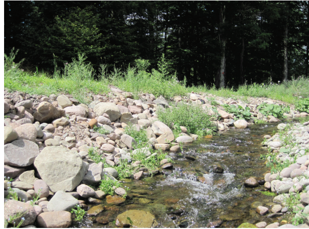
Sloped stone revetment (A1137)
