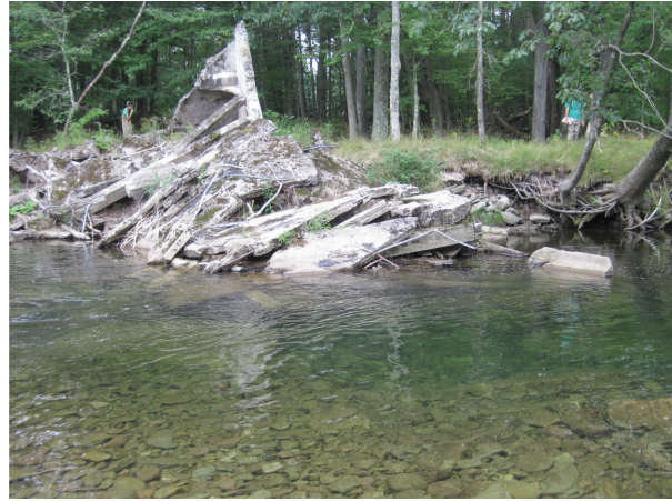
Construction debris (A24)
