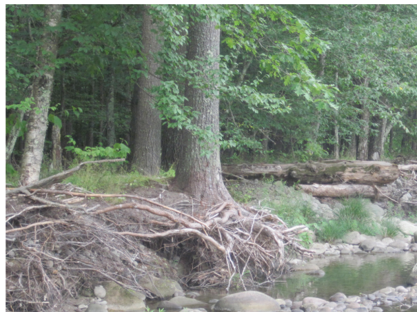
Woody debris jams increasing scour on left bank (B373)
