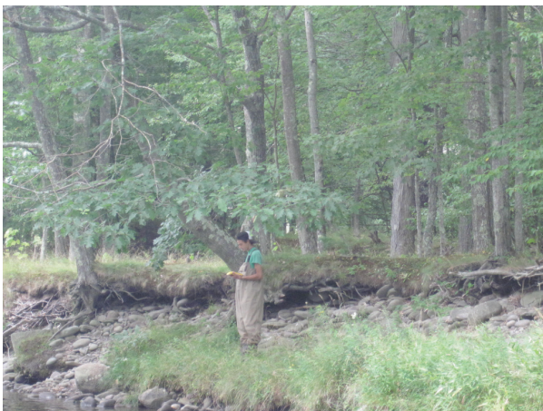
Actively eroding left bank segment (B370)
