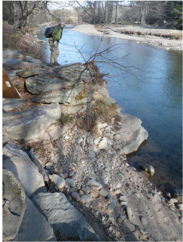
Revetment at Station 19800. (IMG0895)
