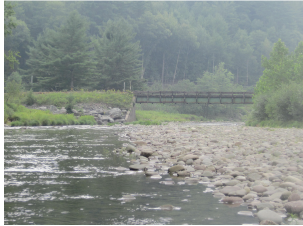
Bridge approach blocking floodplain flow (B474)
