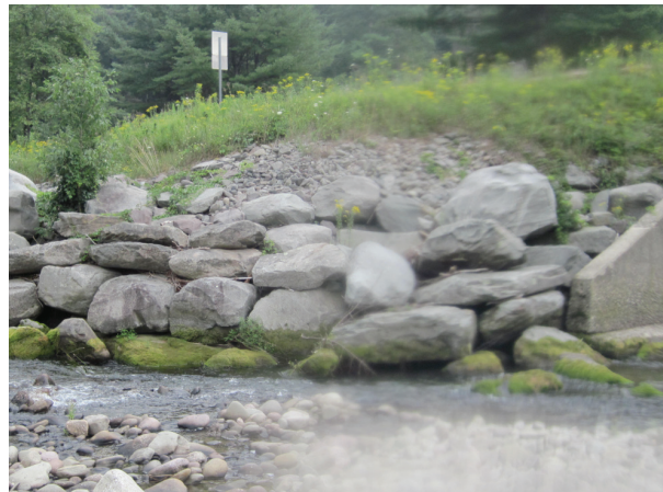
Rip rap revetment upstream of left bank bridge abutments (B476)
