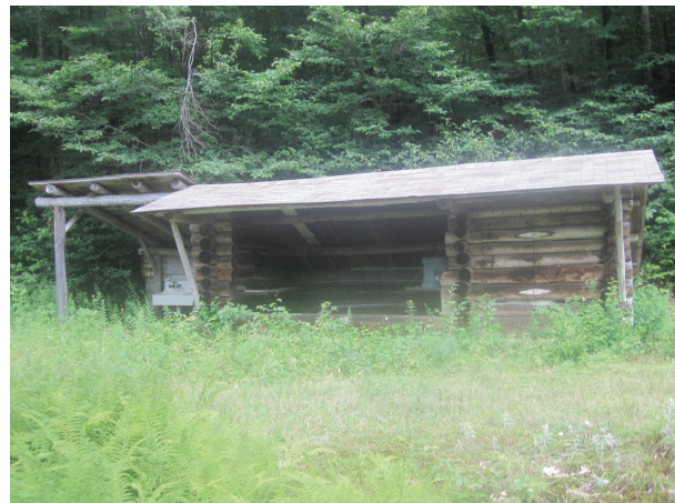
Lean-to on right bank, upslope of revetment (A142)
