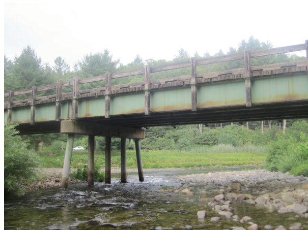
Looking downstream at Hunter Road Bridge (A164)
