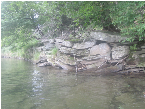
Placed stacked rock revetment on right bank (A140)
