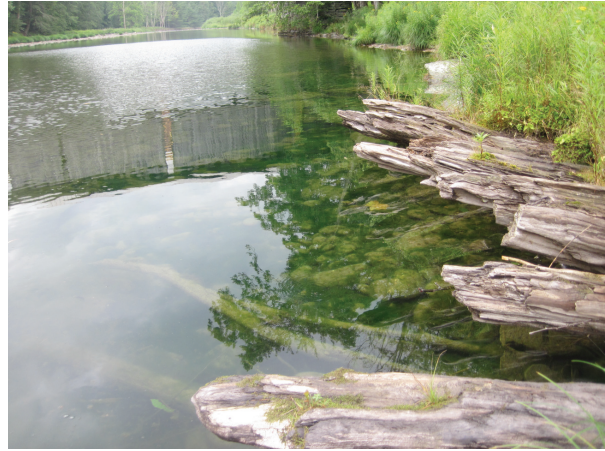
Timber structure creating pool for fish habitat (A182)
