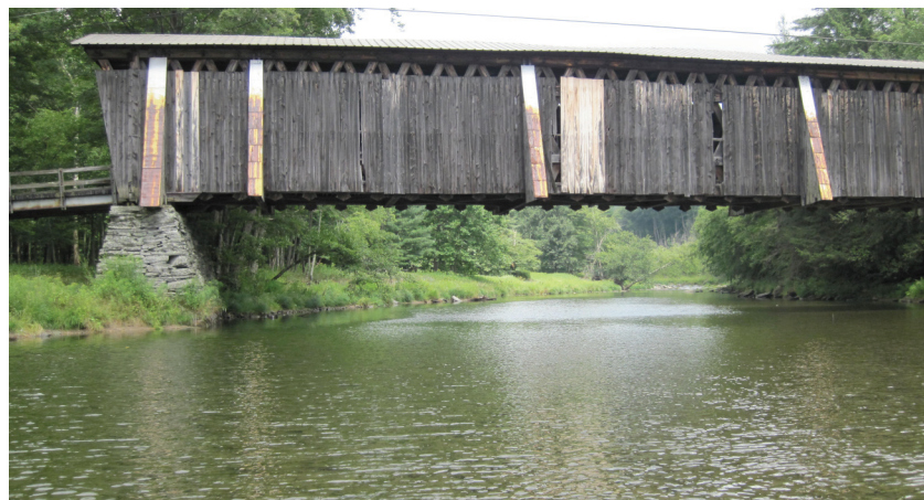
Halls Mills Bridge (B486)
