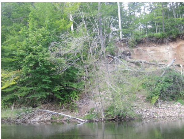
Hydraulic erosion on right bank exposing glacial outwash (A199)
