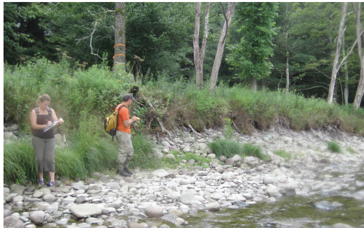
Stabalizing left bank (B488)
