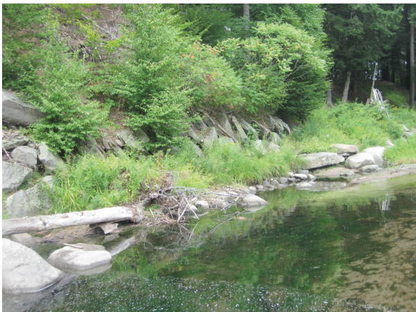
Dumped rock revetment on right bank (A191)
