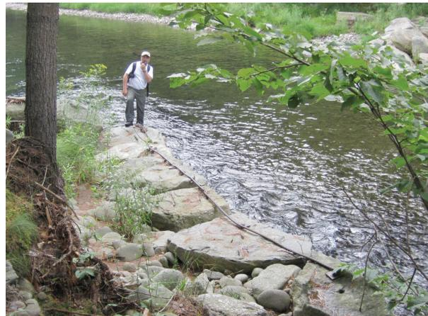
*Stacked rock with pinned rebar on left bank (B495)*
