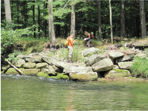
*Slumping revetment due to scour (B497)*
