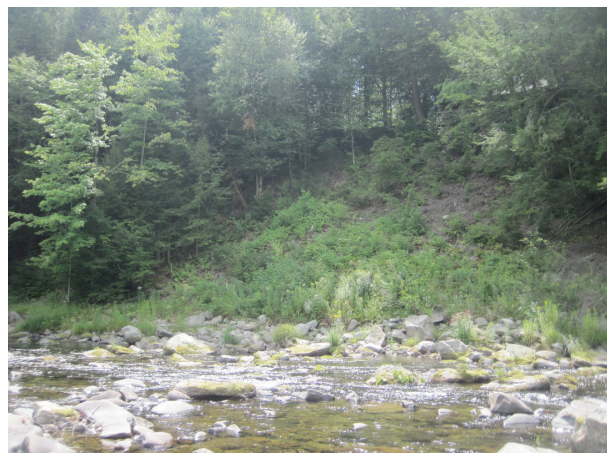
Hydraulic erosion on right bank with hardening at toe (A275)
