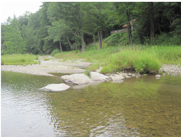
Boulder grade control (A289)
