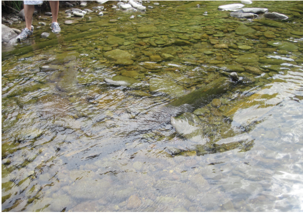
Log cribbing embedded in stream (A294)
