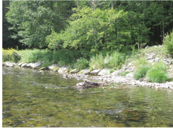
Sloped stone revetment on right bank (A270)
