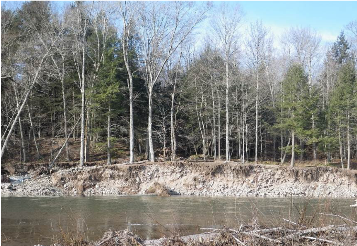
Eroding bank segment on the right bank near Station 27100. (IMG2329)
