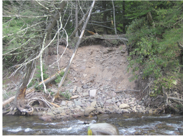
Woody debris causing scour on right bank (A299)
