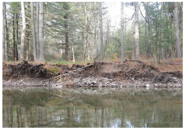
Hydraulic erosion on right bank. (IMPG1689)
