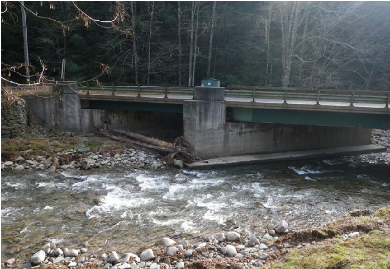
Denning Road Bridge. (IMG1712)
