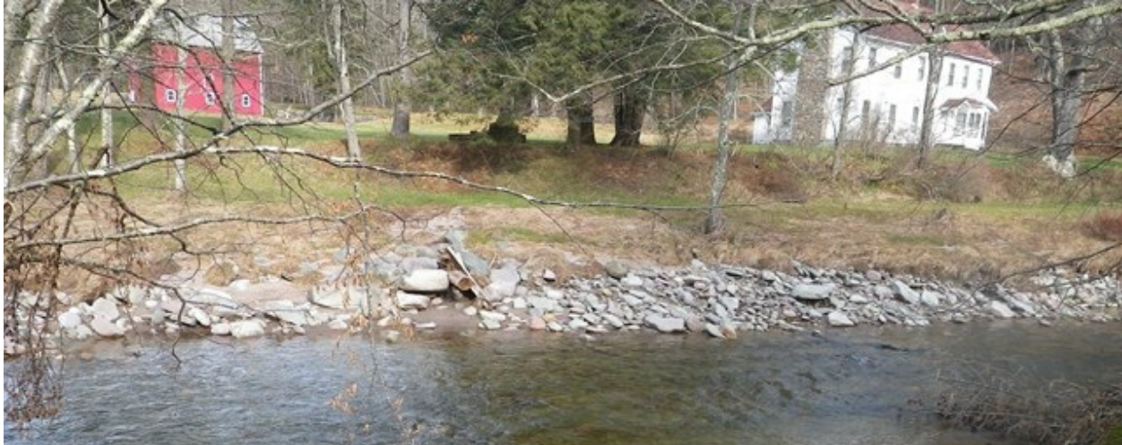
Remnants of wooden dam. (IMGP1686)
