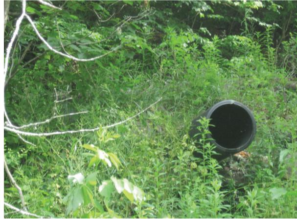
*Plastic culvert conveying road drainage on right bank (B130)*
