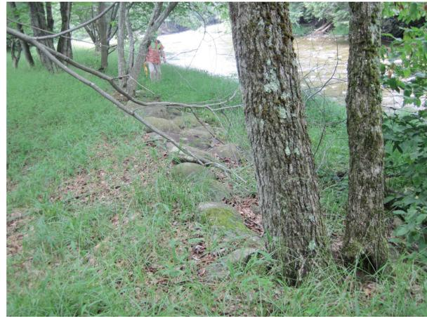
*Washed out stacked rock revetment on left bank (A174)*
