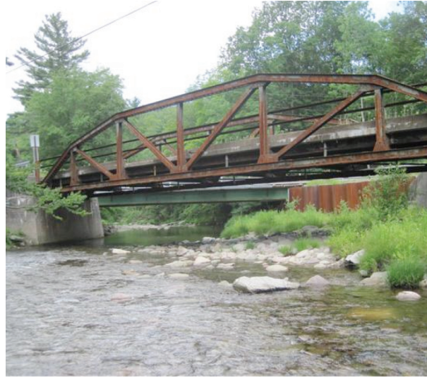
(A304) Denning Road Bridge
