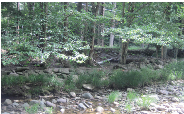
(B257) Cobble stone revetment along right bank
