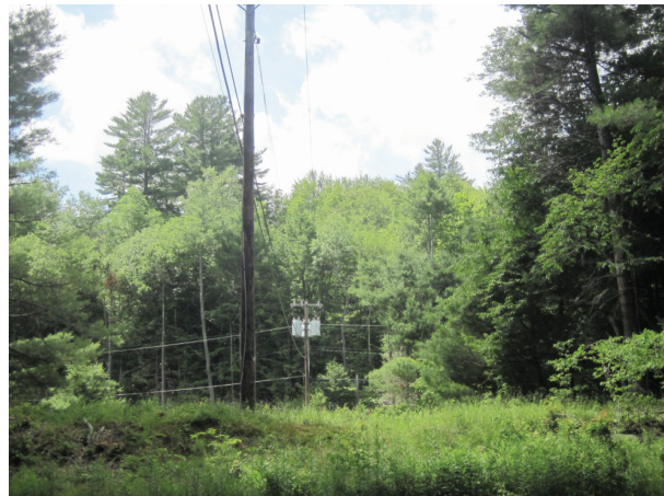
Depositional area in front on berm (B206)
