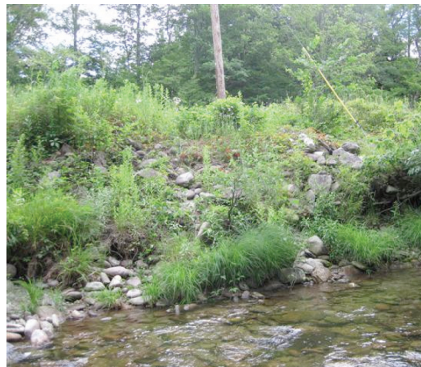
(A315) Rip rap revetment on right bank
