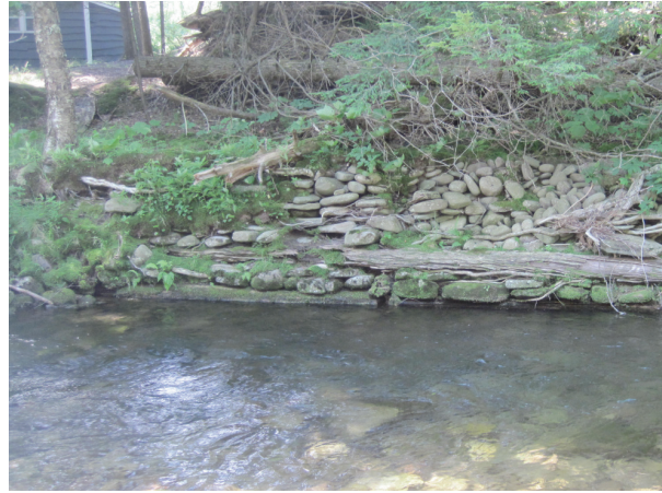
(B248) Cobble and log revetment along left bank
