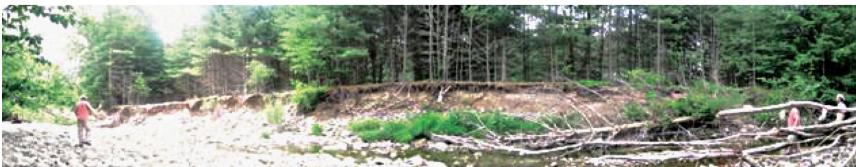
Hydraulic erosion along right bank (A224-229)
