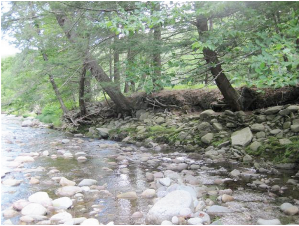
(A284) Erosion on right bank
