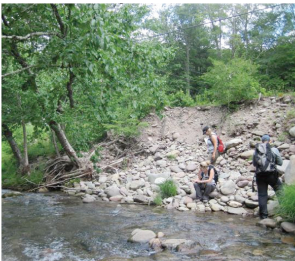
(A298) Erosion along right bank
