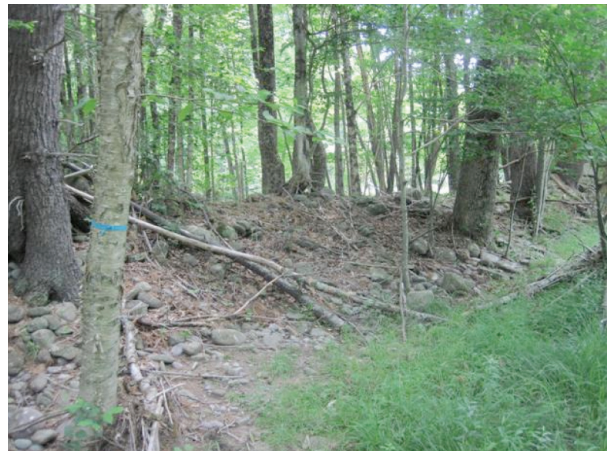
(A267) Old berm on right bank
