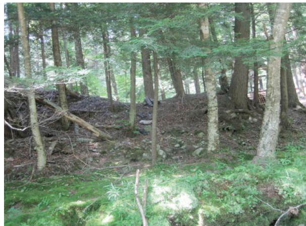
(A262) Berm along left bank
