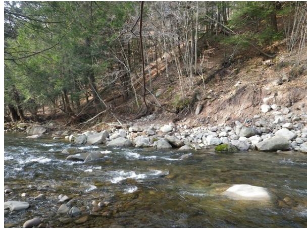
Stabilizing slope failure on the right bank. (IMG1751)
