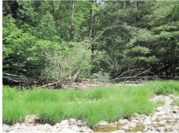
Obstructions along left bank (A416)
