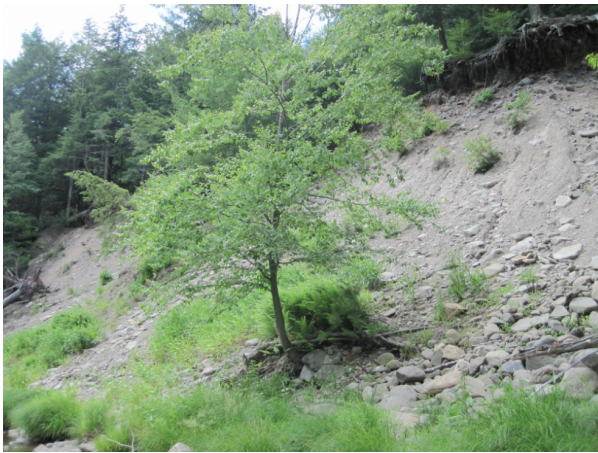
Severe slope failure on right bank (A384)
