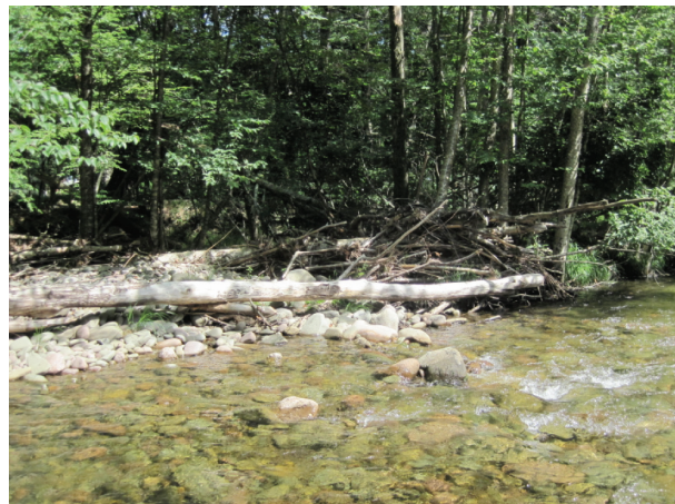
Obstructions along left bank (A418)
