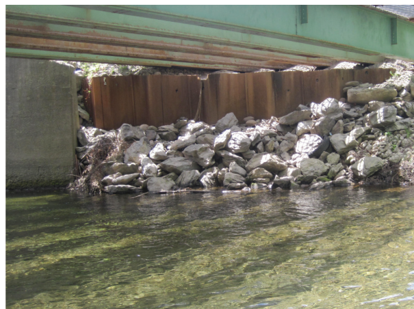
Left bank revetted with rip rap at bridge abutment (B276)
