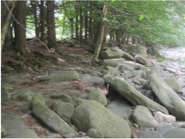
Boulder revetment along left bank (B293)
