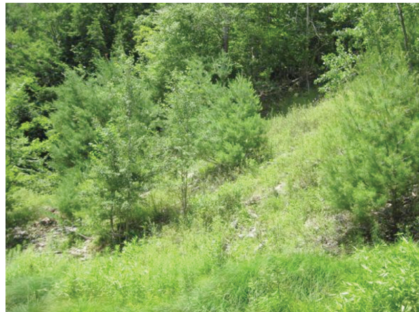
Re-vegetated slope failure (A344)
