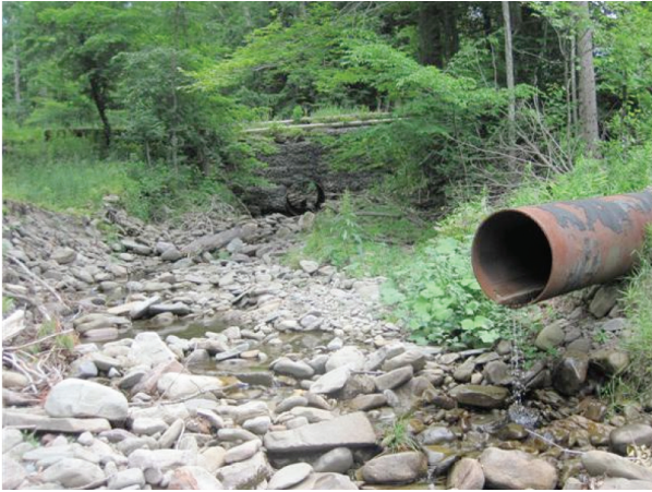
Drainage pipe from Wildcat Road (A313)
