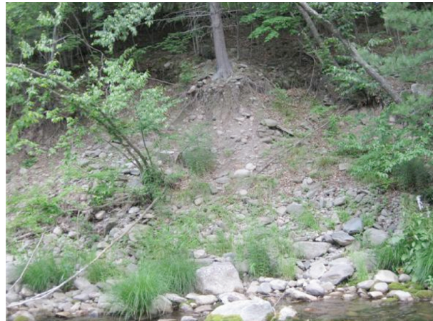
Stabilizing slope failure on right bank (A334)
