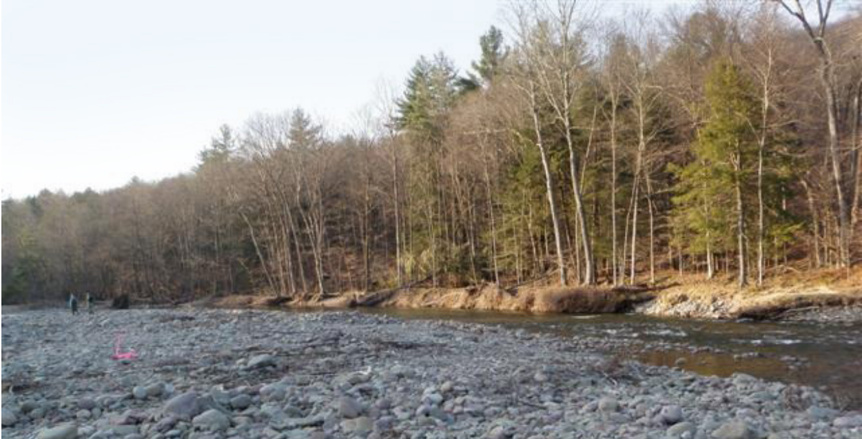
Eroding bank segment on the right bank on the outside of a meander bend. (P1010090)
